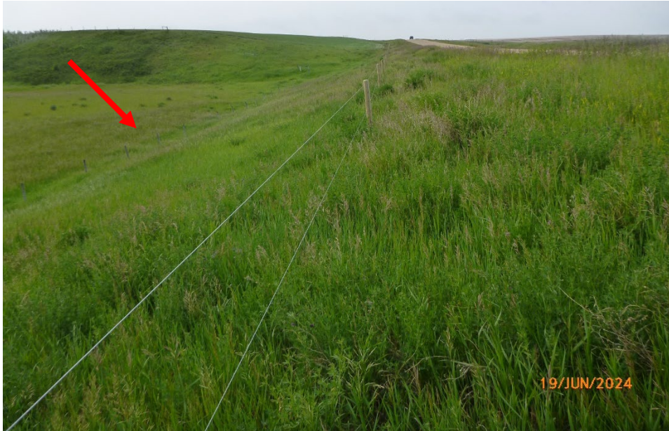
Photo 4 The repaired embankment slope is well vegetated and appears to be in good condition. Photo taken June 19, 2024, facing south.
