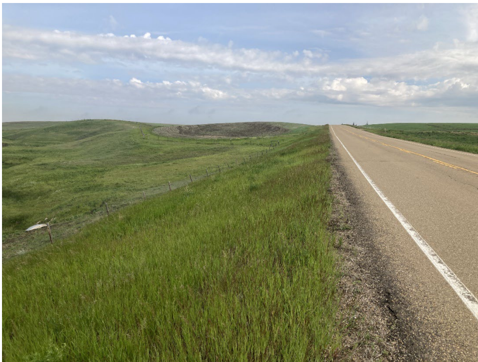
Photo 4 The repaired embankment slope is well vegetated and appears to be in good condition. Photo taken June 19, 2024, facing south.
