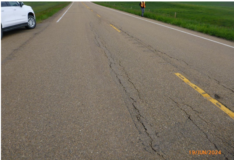
Photo 2 Pavement distress (longitudinal cracking and minor settlement in wheel path) was observed in the west (southbound) lane. Photo take June 19, 2024, facing north.
