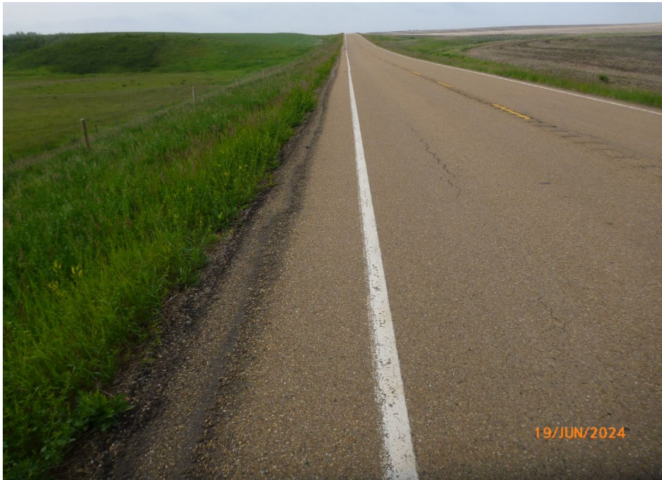
Photo 2 Pavement distress (longitudinal cracking and minor settlement in wheel path) was observed in the west (southbound) lane. Photo take June 19, 2024, facing north.
