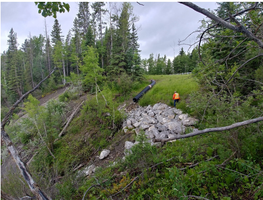
Photo 2 Condition of western slope drain and riprap armouring. Photo taken July 9, 2019 looking northwest.
