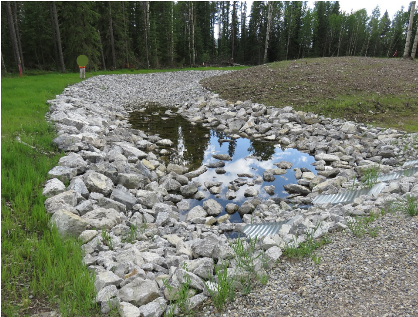
Photo 4 Ponded water at the end of the riprap armoured channel. Photo taken June 12, 2017 looking south.
