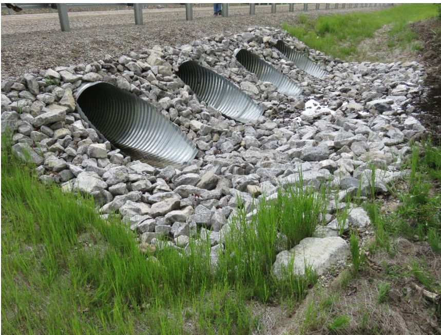
Photo 2 The inlets of the four 1000-mm culverts that were installed in June 2016. Vegetation is growing through the erosion control cloth that was placed around the culverts and in the ditch in June 2016. Photo taken June 12, 2017 looking southwest.
