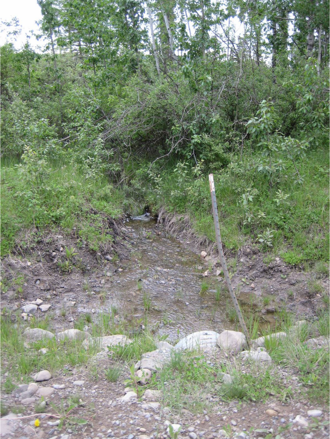
Culvert inlet at south end of site
