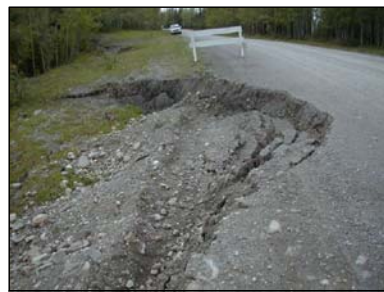
CULVERT OUTLET ~2 m BELOW ROAD (END DISPLACED BY SLIDE) (-SEEPAGE FLOW)
