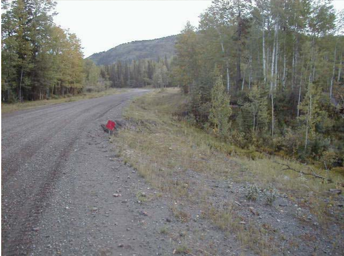
Looking north at upstream end of 600 mm dia culvert
