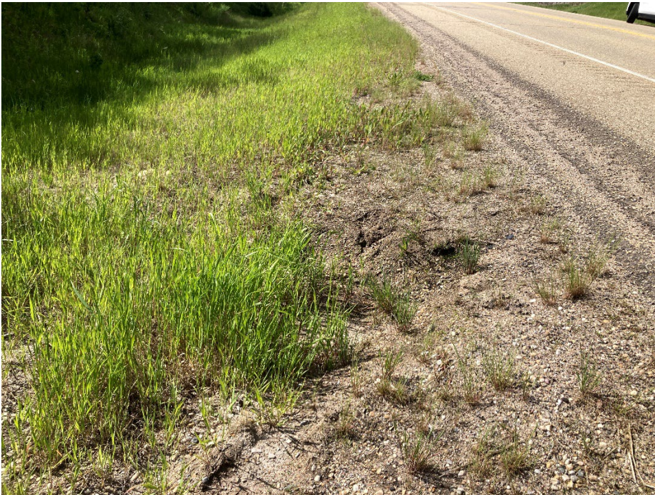
Photo 16 Sinkhole above the culvert in the should of the east (northbound) lane appears similar as during the 2022 inspection. Photo taken June 17, 2024, facing south.
