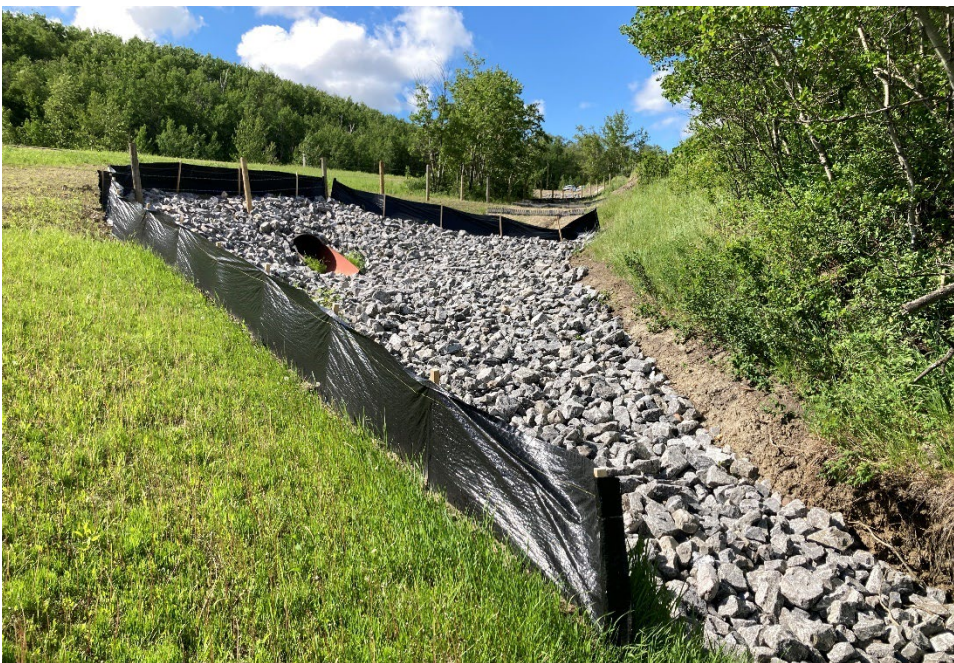
Photo 8 A large riprap apron (Class 1M) was installed in 2023. The riprap apron is over the previous apron and filled the large erosion gully downstream of the culvert outlet. Photo taken June 17, 2024, facing west.
