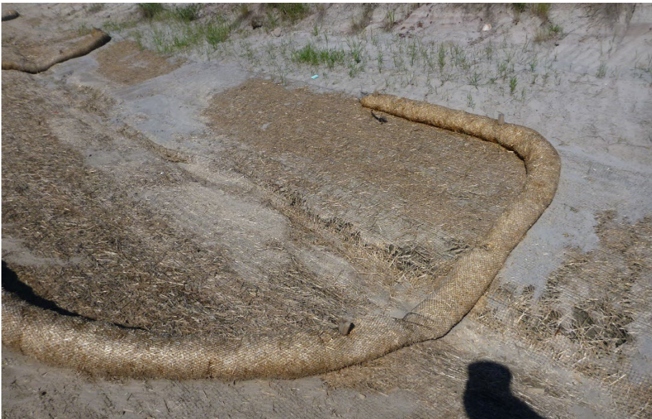
Photo 2 The RECP along portions of the repair is being undermined. Photo taken June 17, 2024, facing north.
