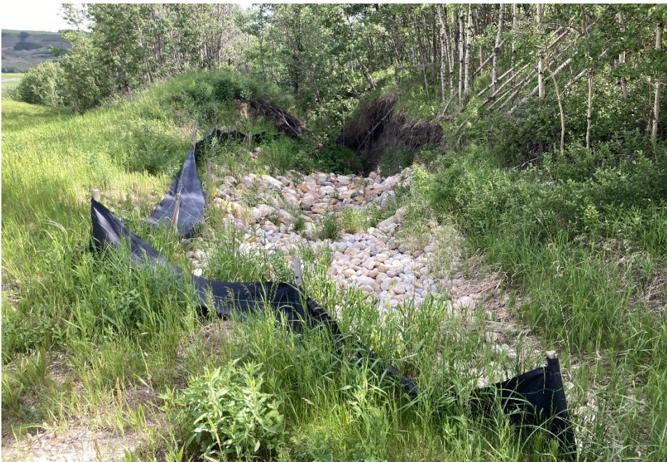
Photo 14 Outlet of culvert and riprap apron at the C075-2 site appears to be in good condition. Photo taken June 17, 2024, facing north.
