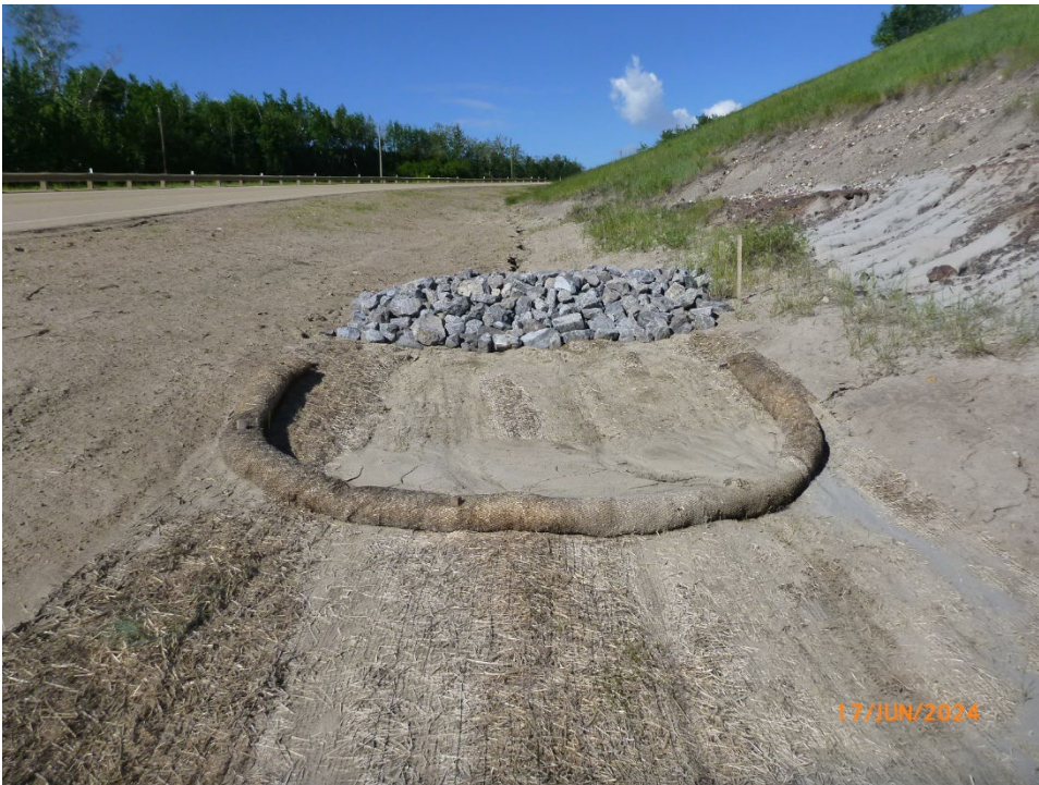
Photo 4 Sediment is accumulating behind the straw wattles. Photo taken June 17, 2024, facing west.
