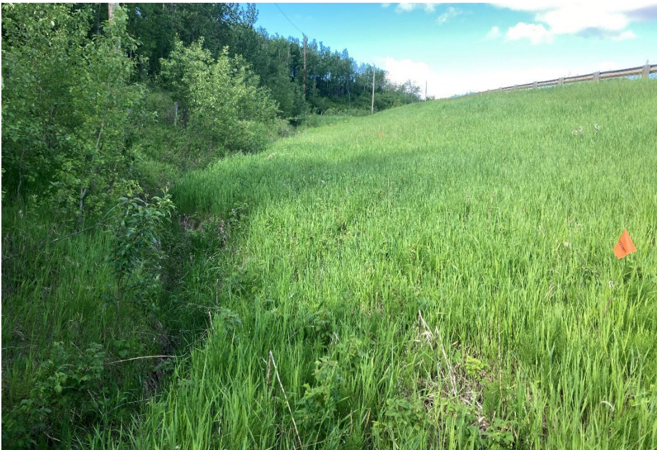
Photo 12 The south highway embankment slope and ditch is well vegetated and appears to be in good condition. Minor ditch erosion in ongoing but is not impacting the highway embankment. Photo taken June 17, 2024, facing west.
