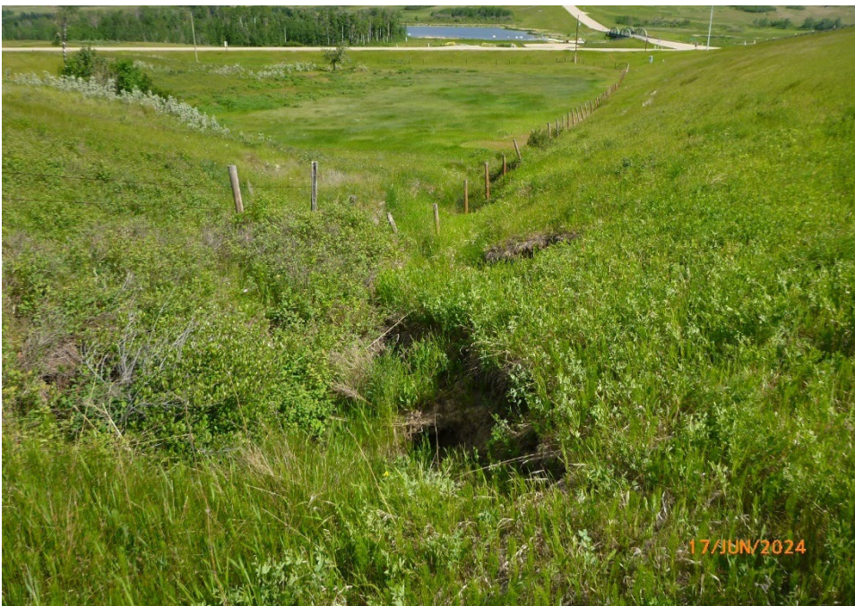
Photo 20 Erosion gully along the toe of the highway embankment (Hwy 609 and Driedmeat Lake in the background). Photo taken June 17, 2024, facing north.
