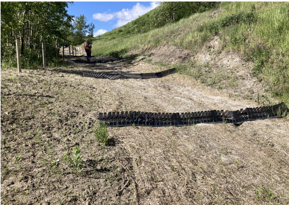
Photo 6 Plastic check dams were installed along the ditch repair, upstream (west) of the culvert outlet. Photo taken June 17, 2024, facing west.
