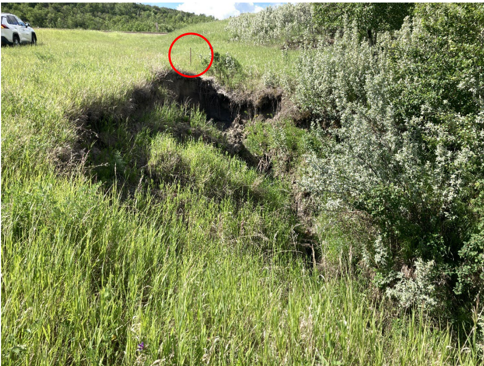
Photo 18 Erosion gully in the west (southbound) ditch along Hwy 56, north of the C075-2 site. Stake installed at upstream end indicated by red circle. Photo taken June 17, 2024, facing south.
