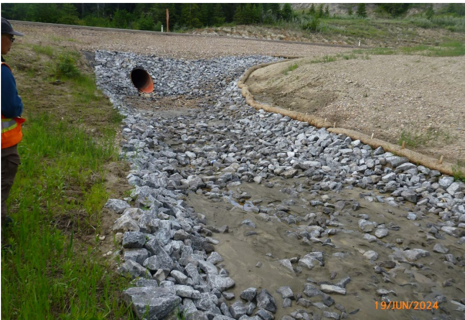
Photo 10 Riprap-lined outlet channel downstream of the culvert underlying Hwy 590. Sediment has been deposited along the channel since late-2023 construction. Photo taken June 19, 2024, facing southwest.
