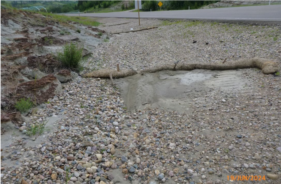
Photo 8 Riprap armoring in the ditch bottom, where the grade of the ditch steepens just west of the culvert outlet underlying Hwy 590. Straw wattles installed along the edge of riprap could direct flows away from riprap and lead to erosion gully formation. Photo taken June 19, 2024, facing east.
