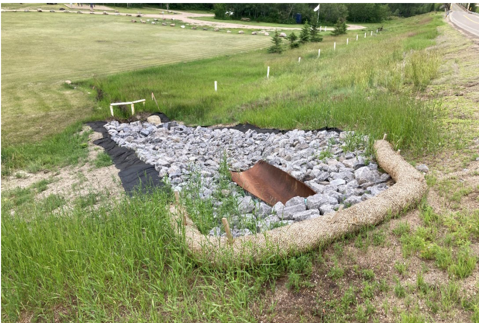
Photo 19 Culvert outlet of new centerline culvert installed in late-2023. Photo taken June 19, 2024, facing southwest.
