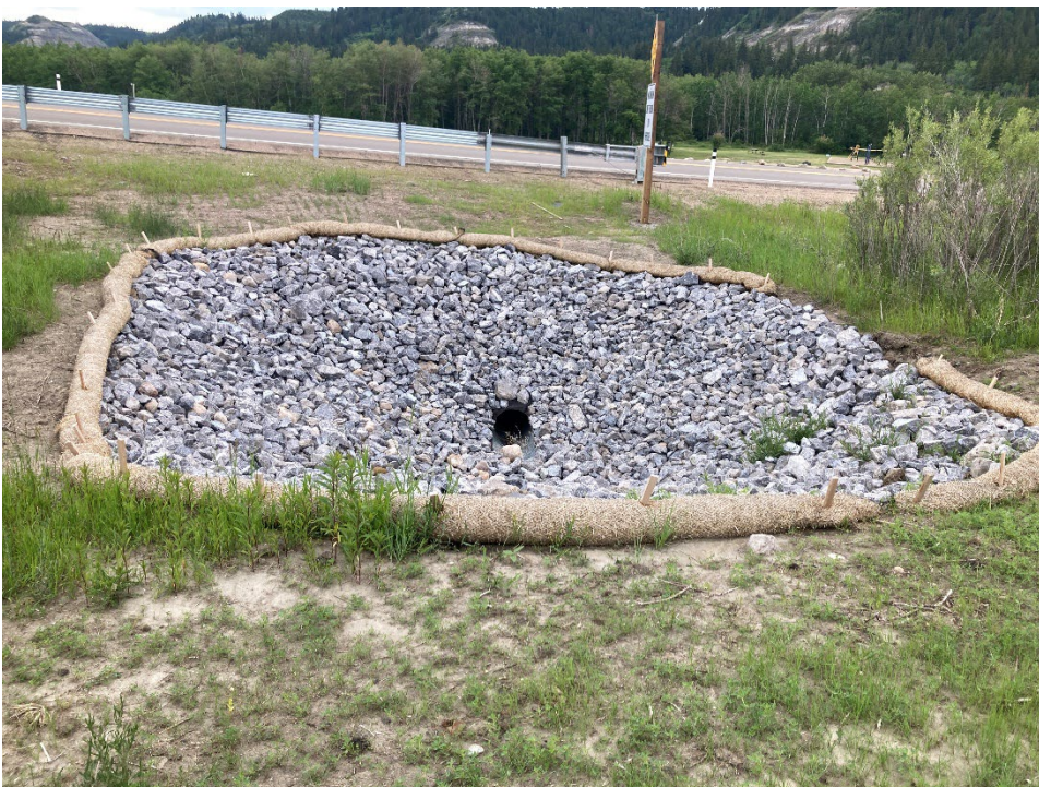
Photo 17 Riprap armoured culvert inlet in the north (westbound) ditch just east of the Red Deer River bridge crossing. Photo taken June 19, 2024, facing southwest.
