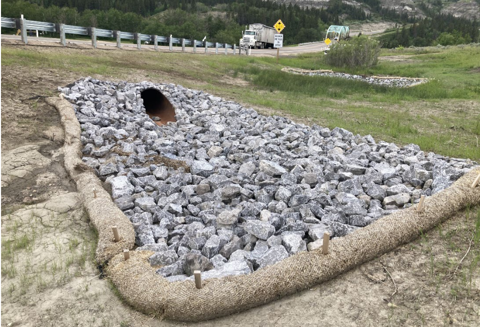
Photo 19 Culvert outlet of new centerline culvert installed in late-2023. Photo taken June 19, 2024, facing southwest.
