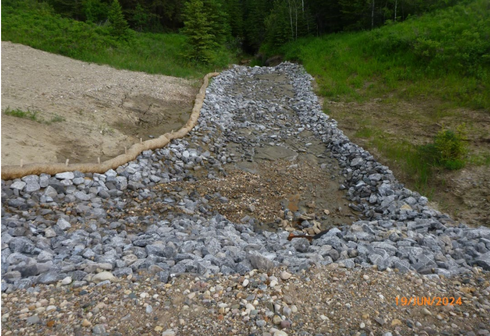
Photo 10 Riprap-lined outlet channel downstream of the culvert underlying Hwy 590. Sediment has been deposited along the channel since late-2023 construction. Photo taken June 19, 2024, facing southwest.
