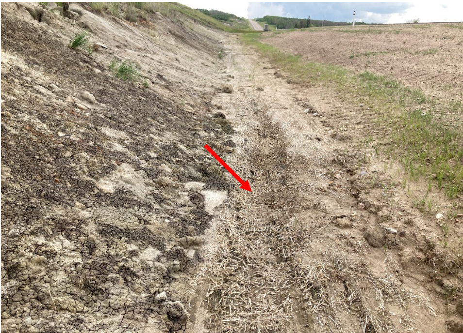
Photo 15 Length of north (westbound) ditch armoured with RECP in late-2023. The RECP is being undermined along the ditch bottom (indicated by red arrow). Photo taken June 19, 2024, facing east.
