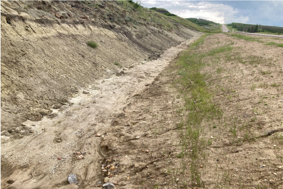
Photo 15 Length of north (westbound) ditch armoured with RECP in late-2023. The RECP is being undermined along the ditch bottom (indicated by red arrow). Photo taken June 19, 2024, facing east.
