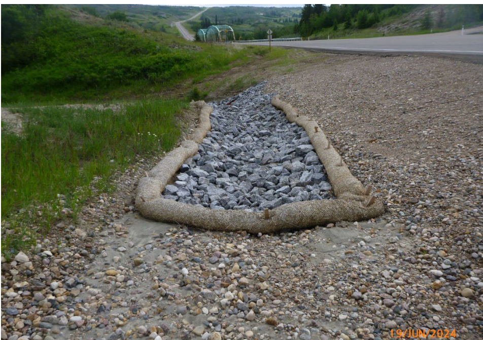
Photo 8 Riprap armoring in the ditch bottom, where the grade of the ditch steepens just west of the culvert outlet underlying Hwy 590. Straw wattles installed along the edge of riprap could direct flows away from riprap and lead to erosion gully formation. Photo taken June 19, 2024, facing east.
