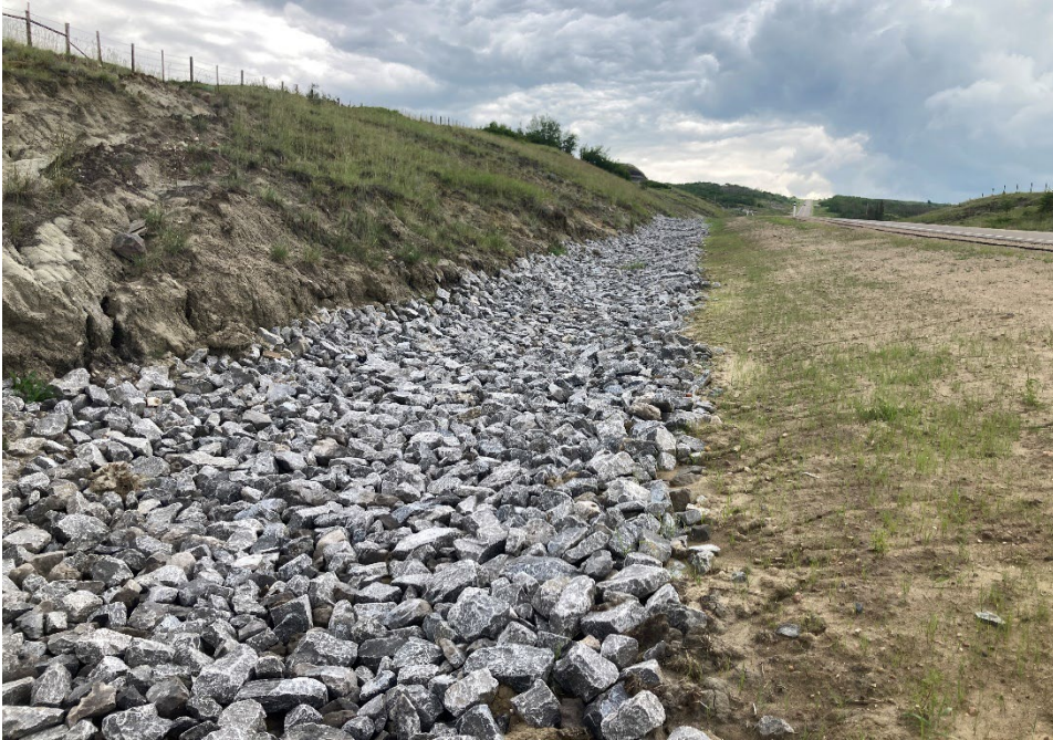
Photo 13 Riprap armouring in the north (westbound) ditch. Photo taken June 19, 2024, facing west.
