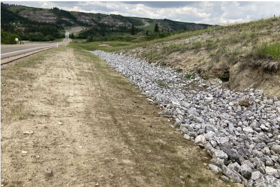
Photo 13 Riprap armouring in the north (westbound) ditch. Photo taken June 19, 2024, facing west.
