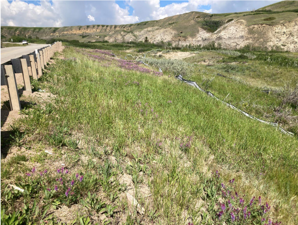
Photo 4 The drain outlet is in good condition. No flow was observed, but there was evidence of recent flow observed at and downstream of the drain outlet. Photo taken June 19, 2024, facing northeast.
