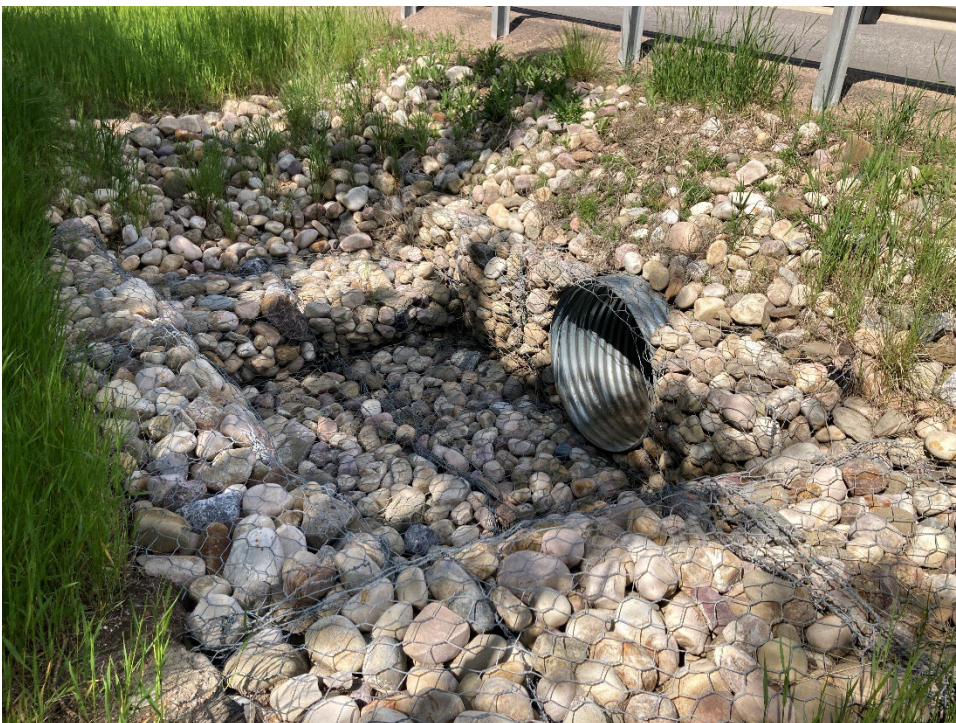
Photo 10 Gabion basket inlet structure appears to be in good condition. Photo taken June 19, 2024, facing northwest.
