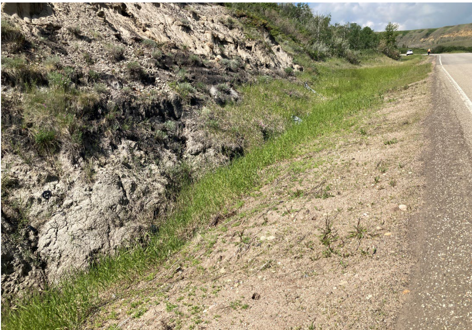
Photo 6 There is ongoing ditch erosion in the south (eastbound) ditch east of the C065-1 subsite (east of the 2021 repair). Photo taken June 19, 2024, facing west.
