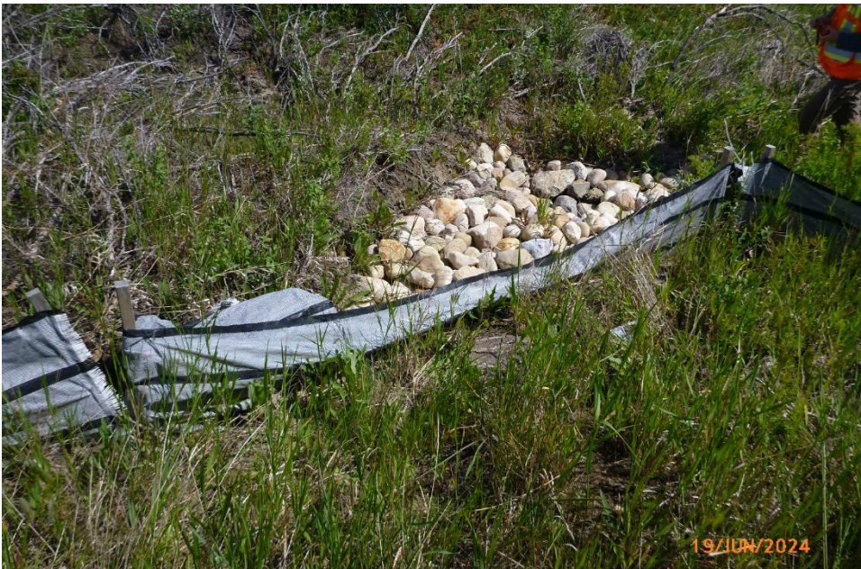
Photo 4 The drain outlet is in good condition. No flow was observed, but there was evidence of recent flow observed at and downstream of the drain outlet. Photo taken June 19, 2024, facing northeast.
