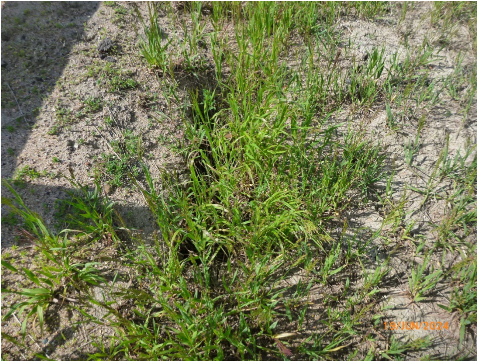
Photo 14 Settlement of fill above the 2021 H-pile wall. Photo taken June 19, 2024, facing west.
