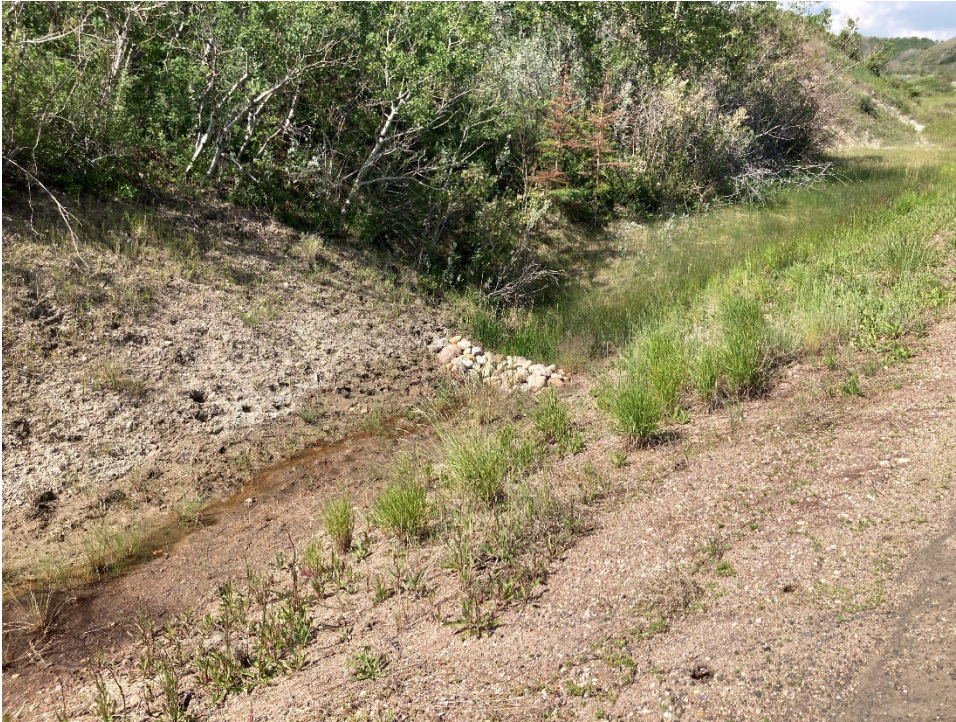
Photo 6 There is ongoing ditch erosion in the south (eastbound) ditch east of the C065-1 subsite (east of the 2021 repair). Photo taken June 19, 2024, facing west.
