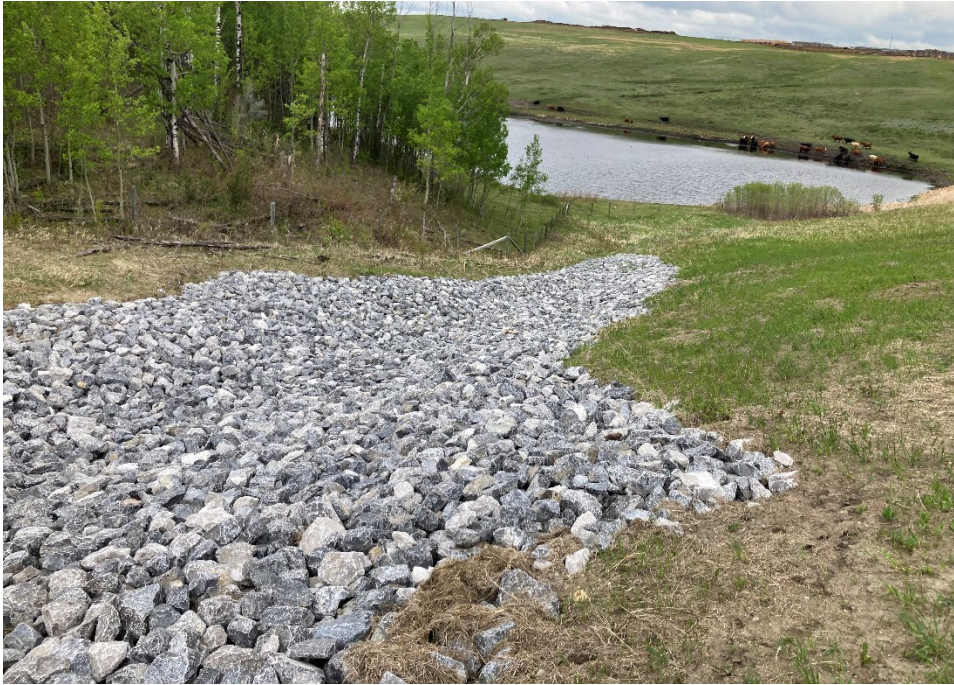
Photo 8 The backfilled erosion gully near the top of the slope. Photo taken May 30, 2022, facing southwest.
