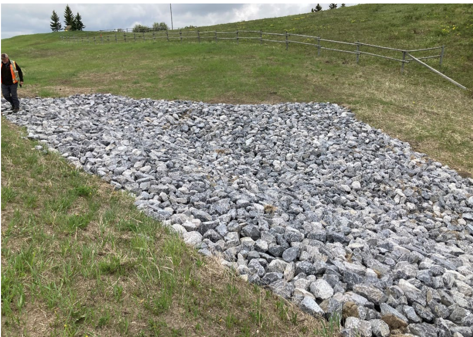
Photo 8 The backfilled erosion gully near the top of the slope. Photo taken May 30, 2022, facing southwest.
