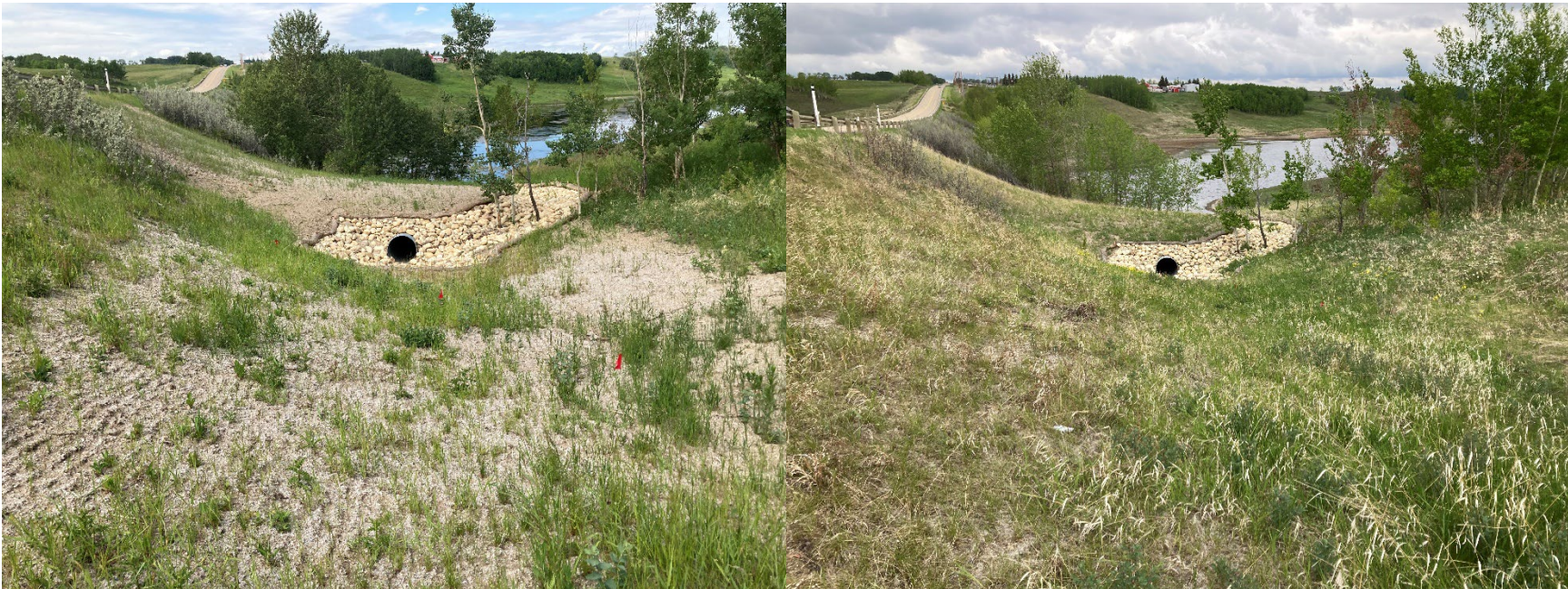
Photo 1 The vegetation cover in the north (westbound) ditch and repaired slope has increased significantly since the 2021 inspection. Photos taken June 23, 2021 and May 30, 2022, facing west.
