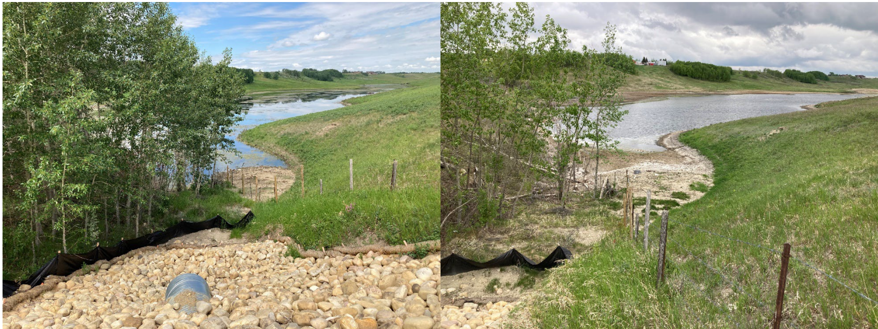
Photo 2 The Carstairs Creek water level has decreased by 0.5 m to 1.0 m between the 2021 and 2022 inspections. Photo taken June 23, 2021 and May 30, 2022, facing northwest.
