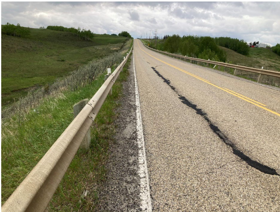
Photo 6 Pavement cracking in the eastbound lane, west of the C073-I site that was repaired in August 2020. Photo taken May 30, 2022, facing west.
