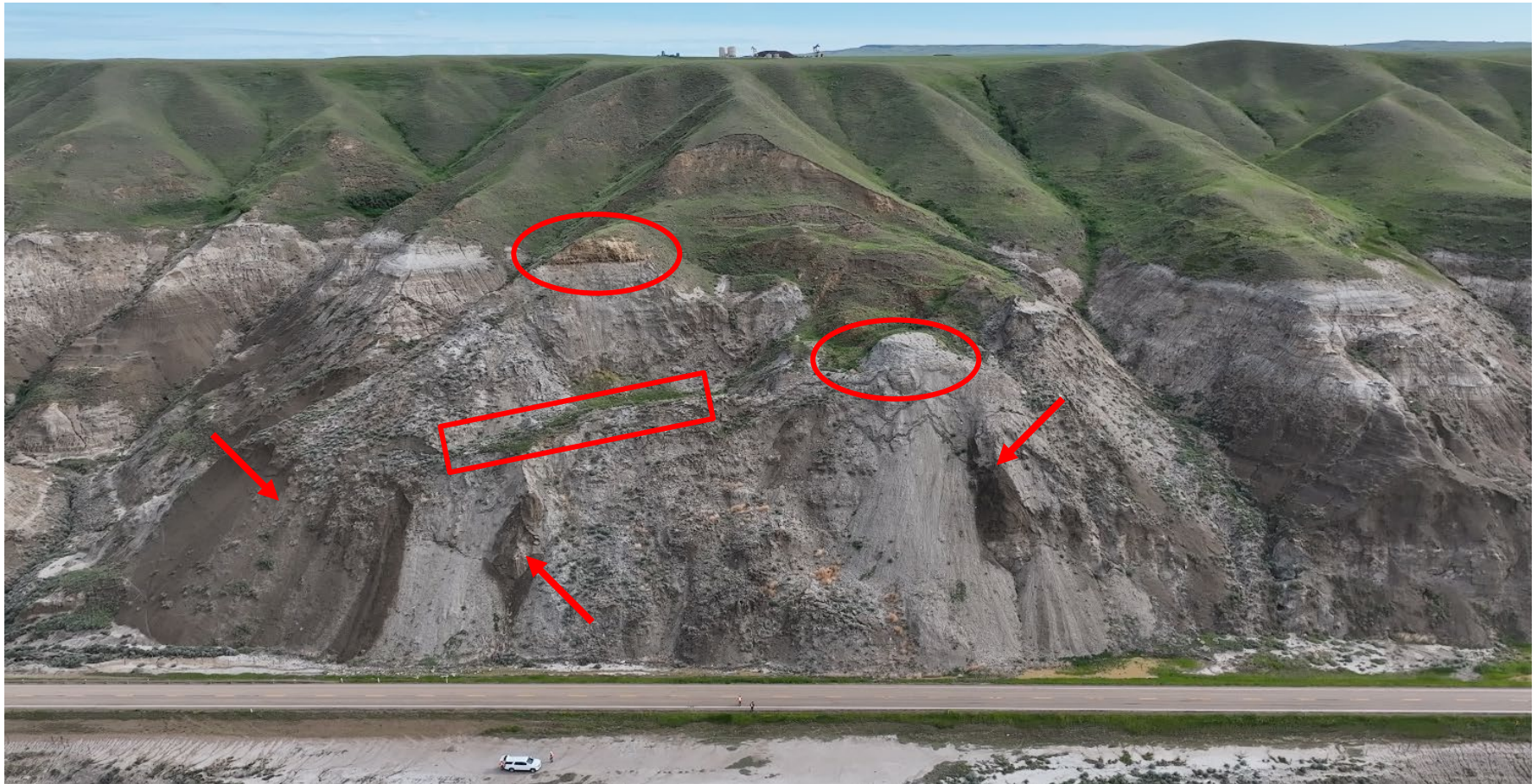
Photo 1 Aerial photo of the C077 site. Locations of recent movement are indicated by red arrows, location of new (late-2023 or early-2024) ground cracking observed on the slope is indicated by red rectangle, and previous scaling completed in 2022 is indicated by red circles (note the area of ground cracking was also scaled in 2022). Photo taken June 18, 2024, facing north.
