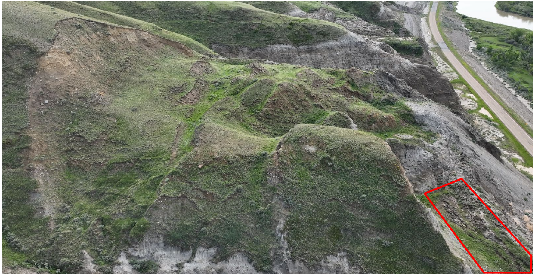
Photo 5 Aerial view of the top portion of the slide. Area of new ground cracks indicated by red polygon. Photo taken June 18, 2024, facing east.
