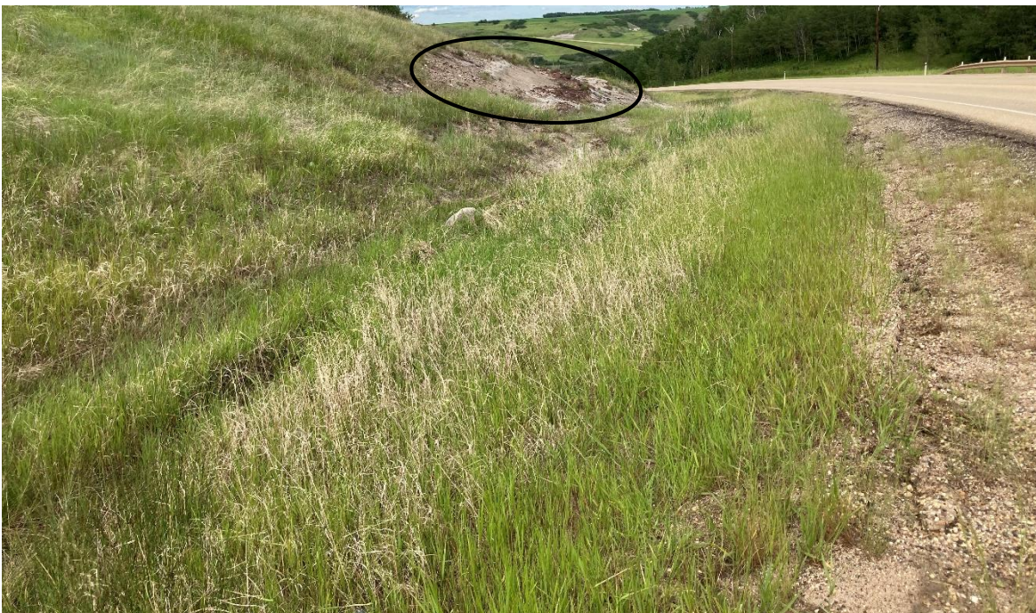
Photo 10 The ditch is well vegetated upslope (northwest) of the bedrock outcrop (indicated by black ellipse). Photo taken June 24, 2020 facing southeast.
