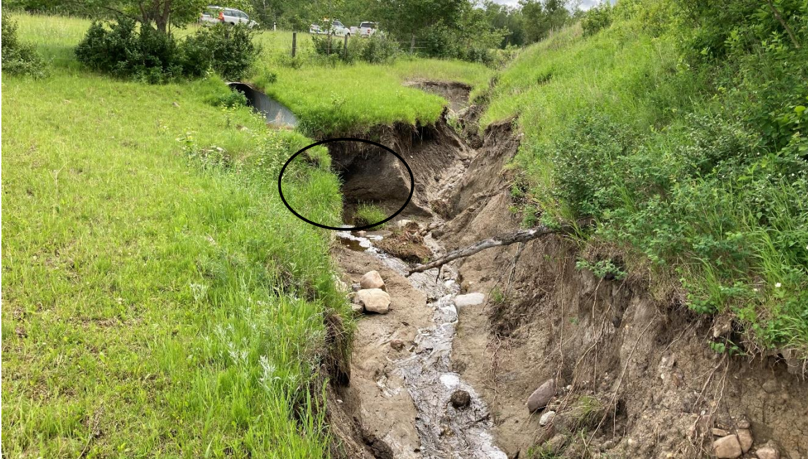
Photo 4 Erosion upslope of the culvert outlet that is impacting the existing fence. Photo taken June 24, 2020 facing northeast.
