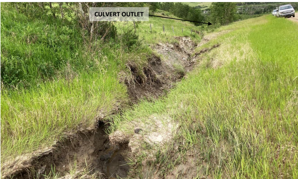
Photo 8 Erosion upslope of the culvert outlet. The approximate location of the culvert outlet is indicated by the black arrow. Photo taken June 24, 2020 facing northeast.
