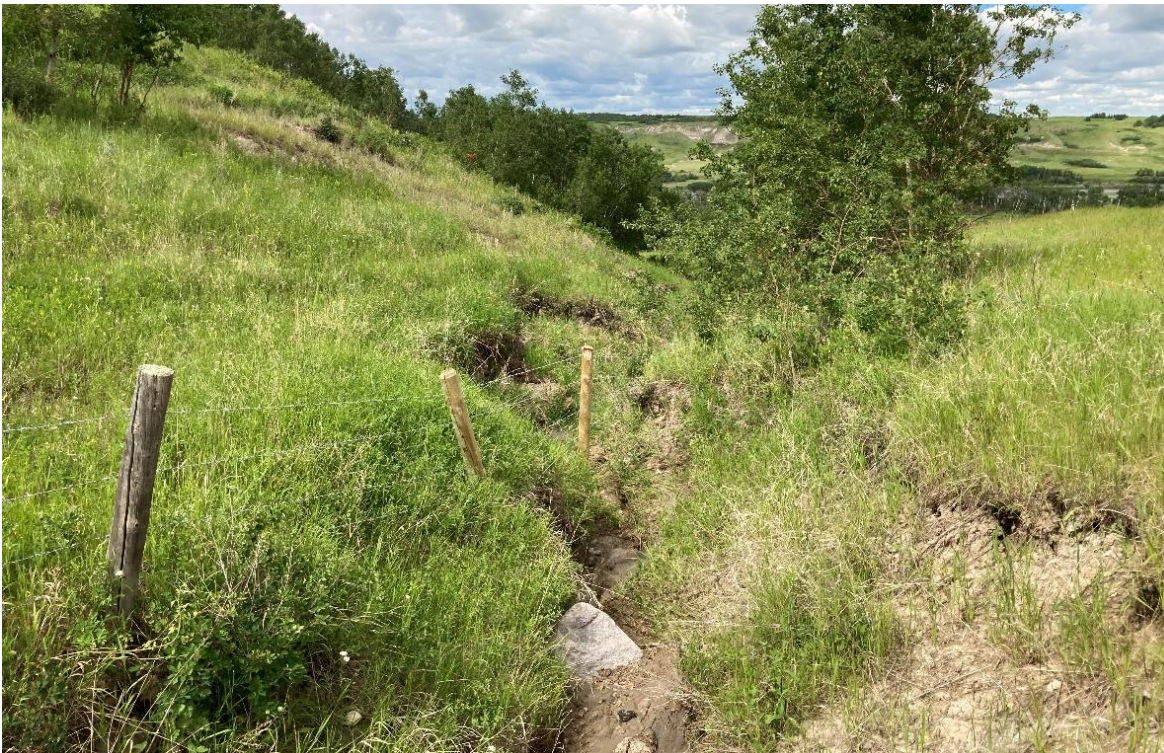
Photo 4 Erosion upslope of the culvert outlet that is impacting the existing fence. Photo taken June 24, 2020 facing northeast.
