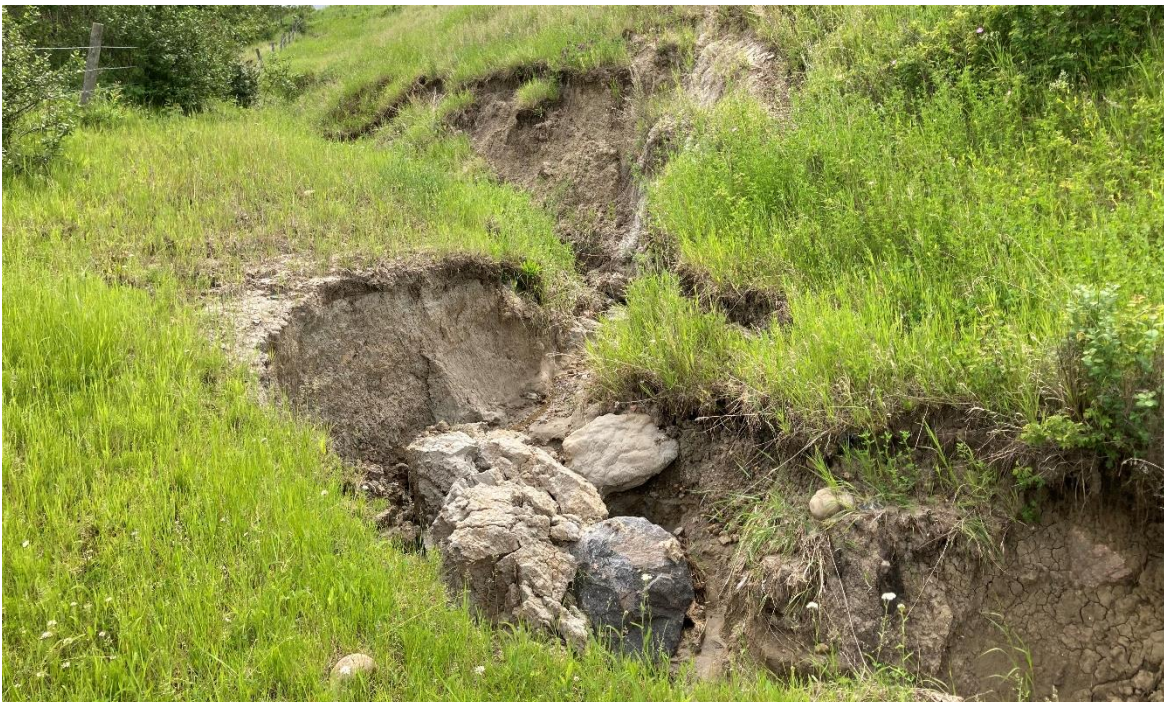
Photo 6 Erosion increasing in depth upslope of the culvert outlet. Photo taken June 24, 2020 facing southwest.
