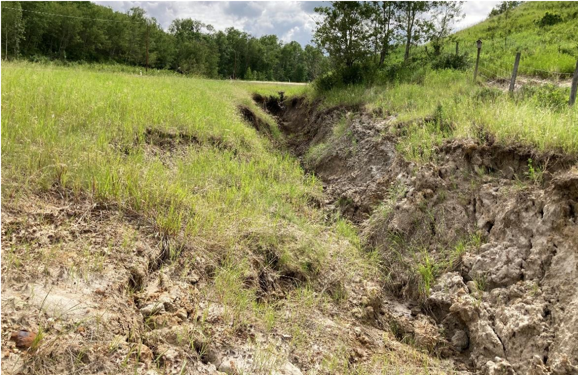
Photo 6 Erosion increasing in depth upslope of the culvert outlet. Photo taken June 24, 2020 facing southwest.
