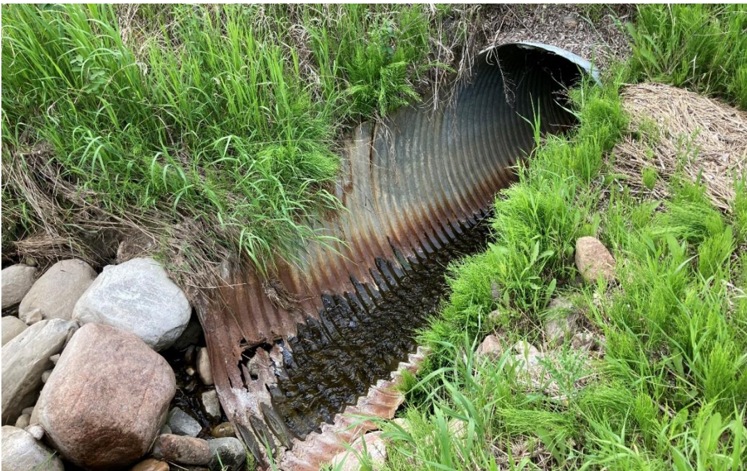
Photo 2 Culvert inlet. The bottom of the culvert is corroded and water is leaking into the underlying material. Photo taken June 24, 2020 facing north.
