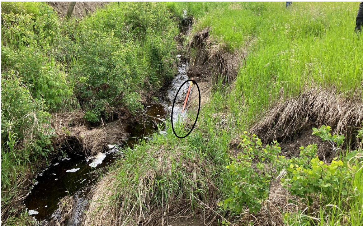
Photo 12 Erosion on the south side of Hwy 609:02 has exposed an underground utility line (indicated by black ellipse). Photo taken June 24, 2020 facing west.
