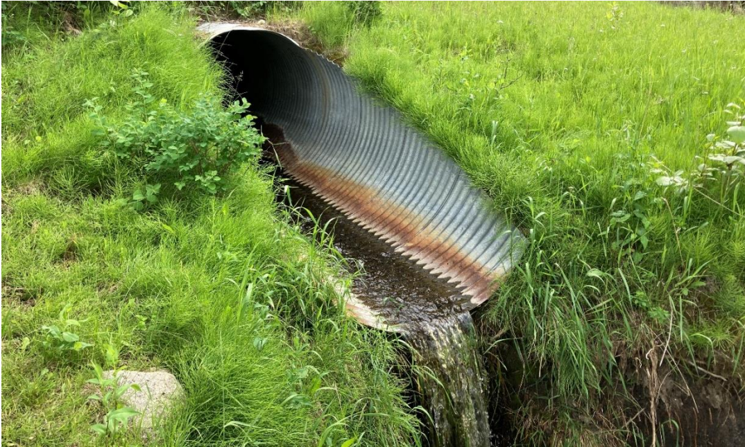
Photo 2 Culvert inlet. The bottom of the culvert is corroded and water is leaking into the underlying material. Photo taken June 24, 2020 facing north.
