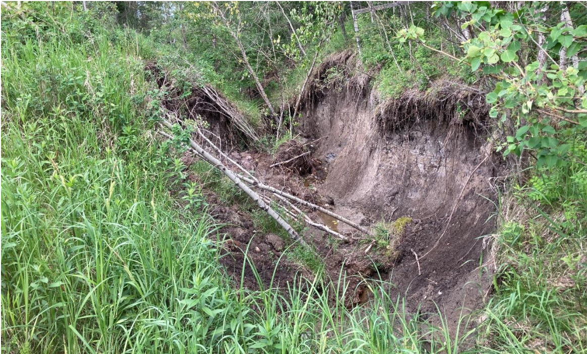
Photo 16 Outlet of the erosion gully on the east side of Hwy 56:16 (southeast of C054). Photo taken June 24, 2020 facing south.
