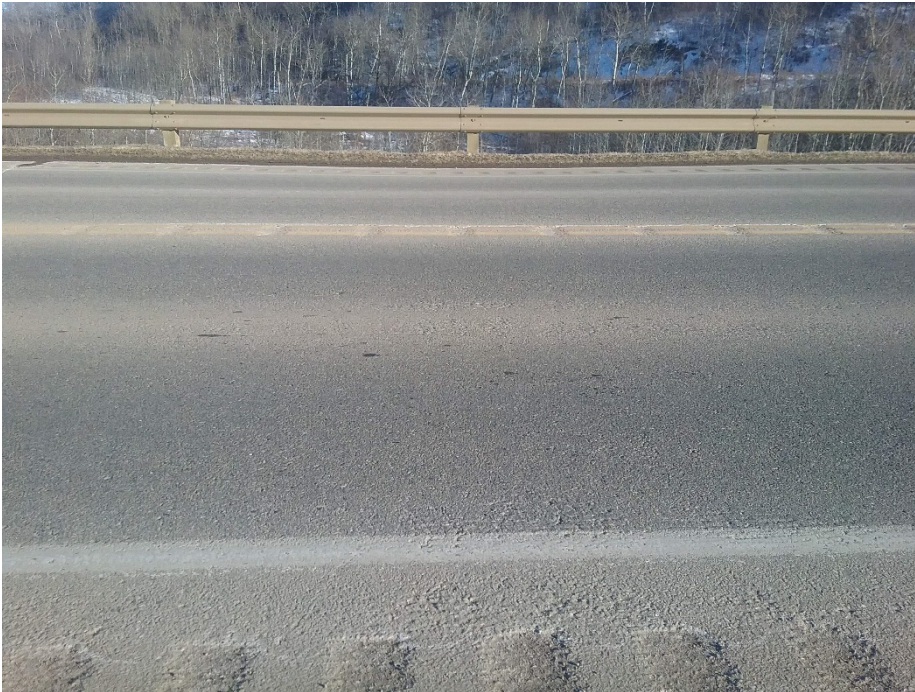
Photo 4 Transverse pavement crack extending entire width of highway. Photo taken on February 28, 2018.
