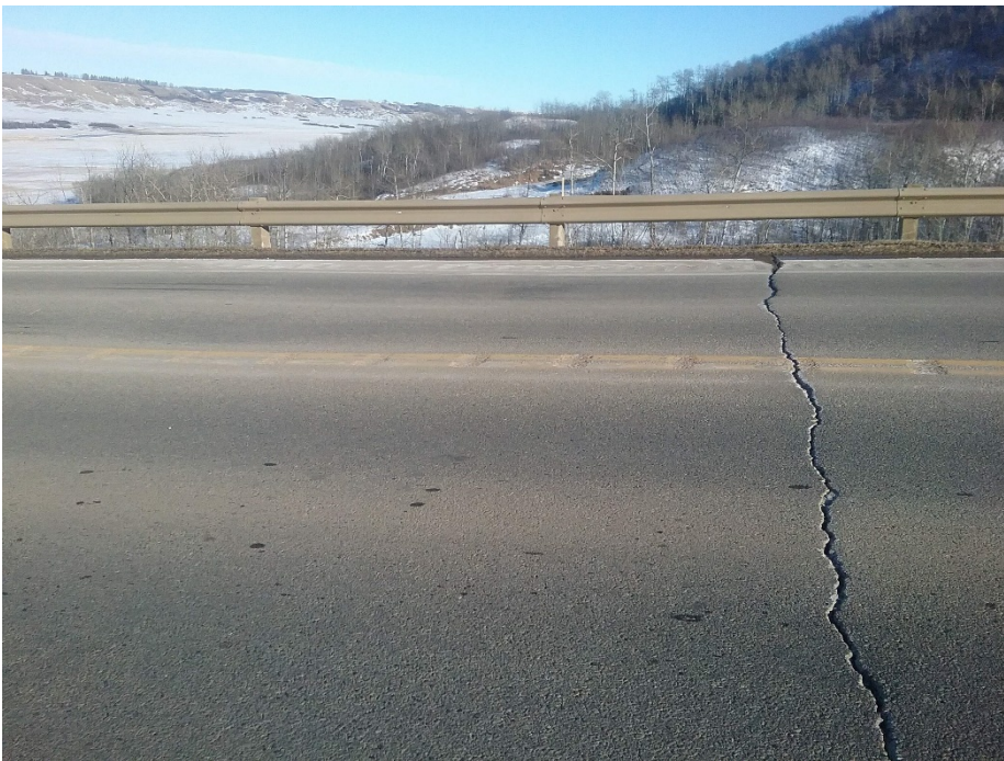
Photo 2 Minor pavement depression on northbound lane and transverse pavement cracking south of depression. Photo taken on February 28, 2018 looking east.
