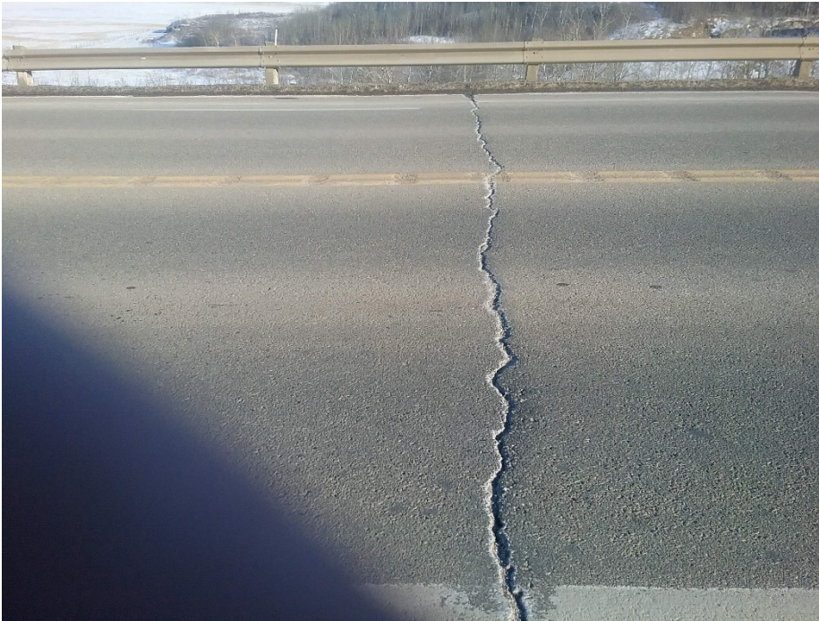
Photo 2 Minor pavement depression on northbound lane and transverse pavement cracking south of depression. Photo taken on February 28, 2018 looking east.
