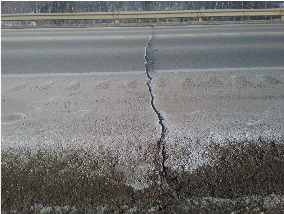
Photo 4 Transverse pavement crack extending entire width of highway. Photo taken on February 28, 2018.
