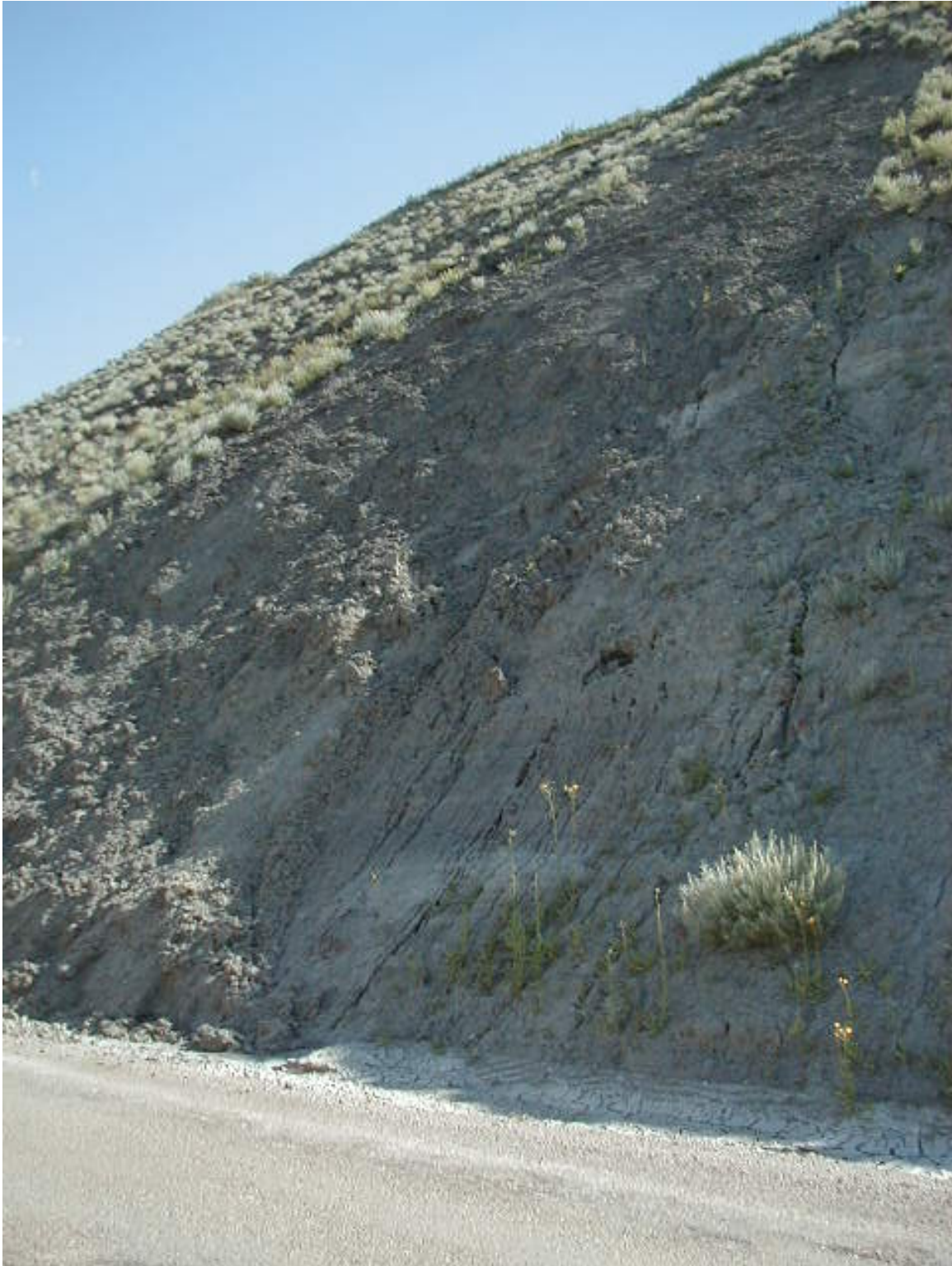
Backslope Erosion
