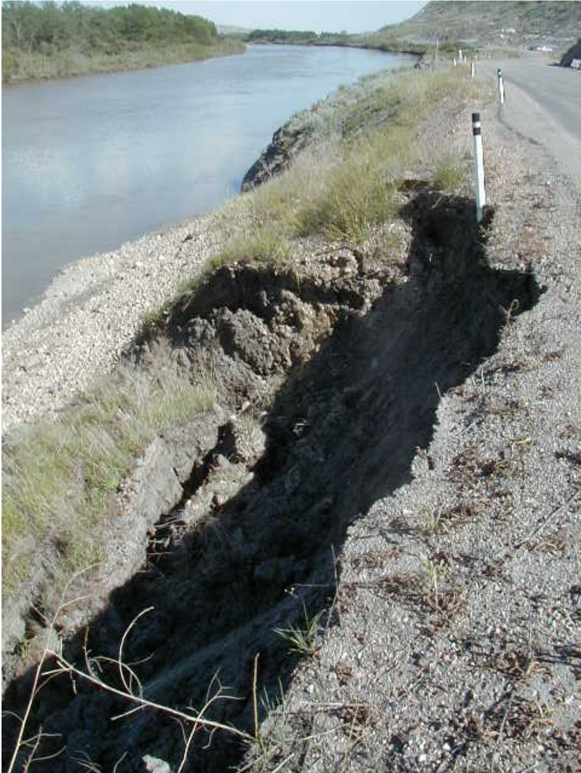
View of new slump section at north end of gravel berm due to June 2005 flooding. Width is about 13 m.
