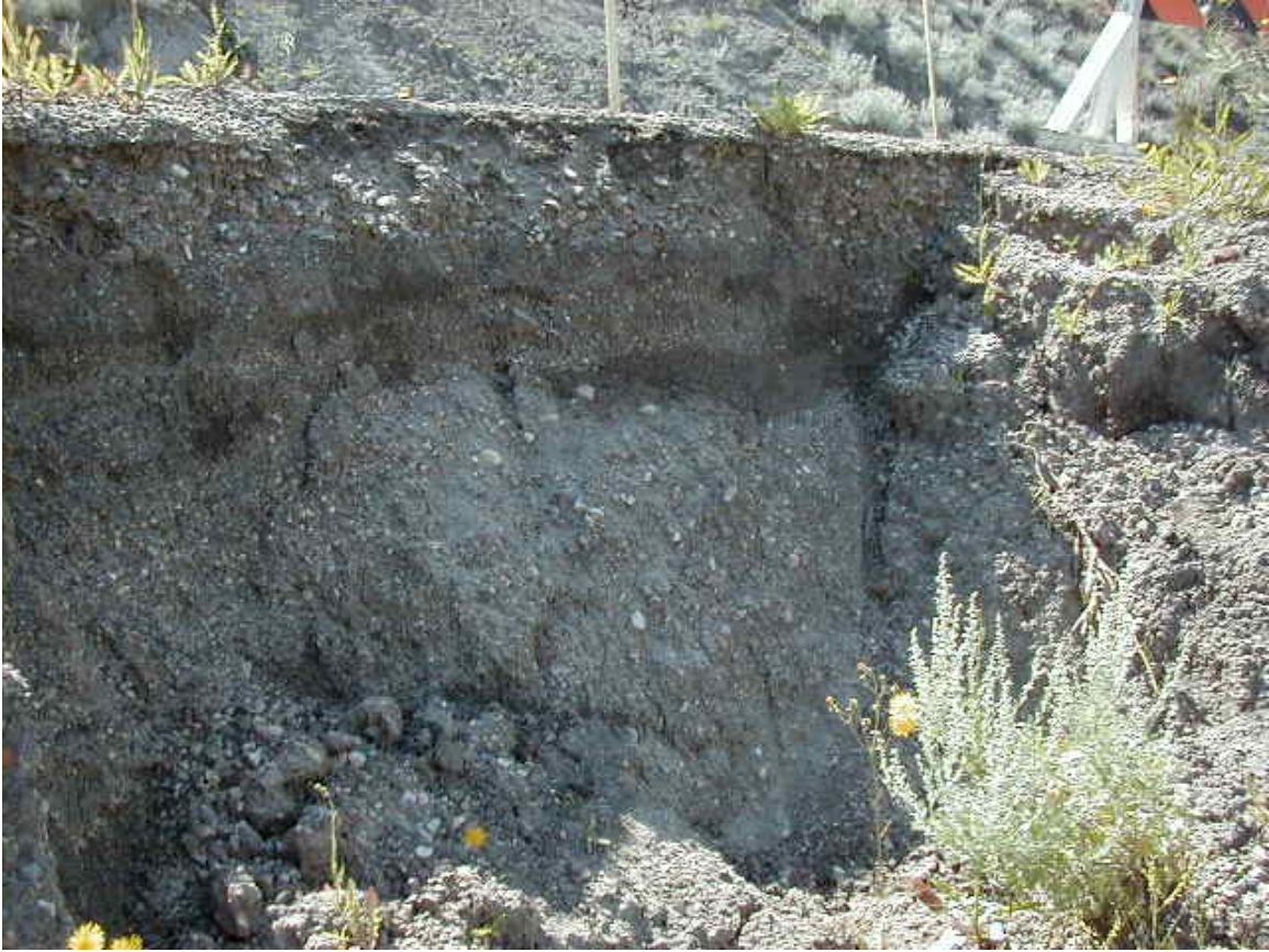
Another view of the main scarp next to the highway.
