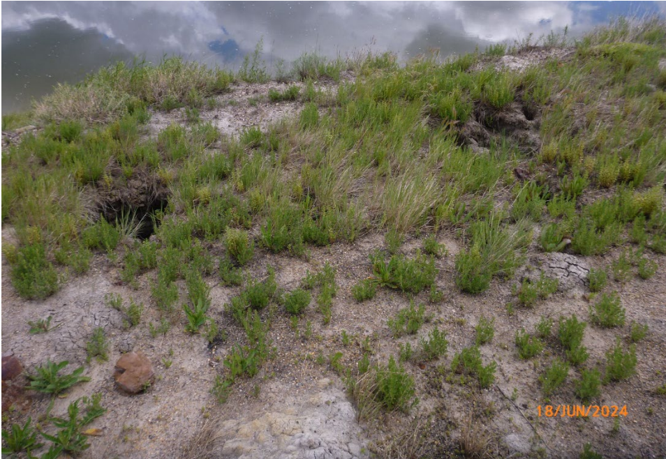
Photo 10 Sinkhole observed in the highway embankment slope downslope of C018-2. Photo taken June 18,2024, facing north.
