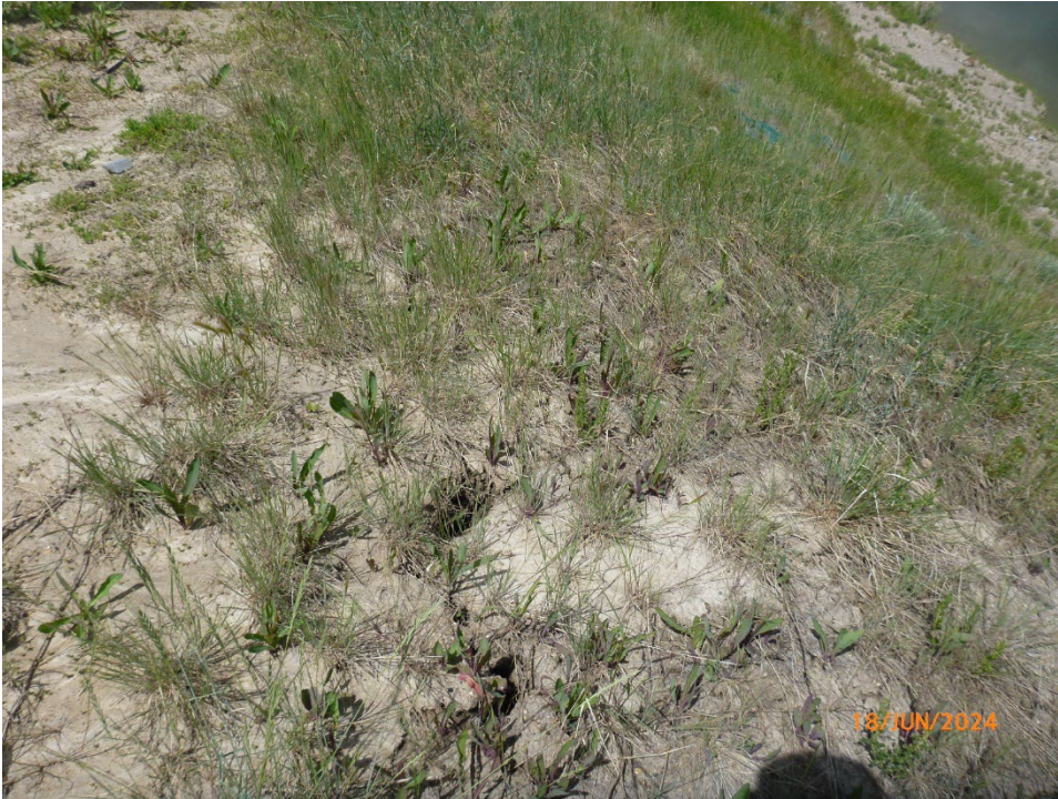
Photo 8 Sinkhole observed in the highway embankment slope downslope of C018-2. Photo taken June 18, 2024, facing north.
