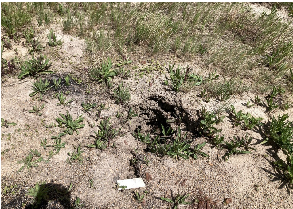
Photo 8 Sinkhole observed in the highway embankment slope downslope of C018-2. Photo taken June 18, 2024, facing north.
