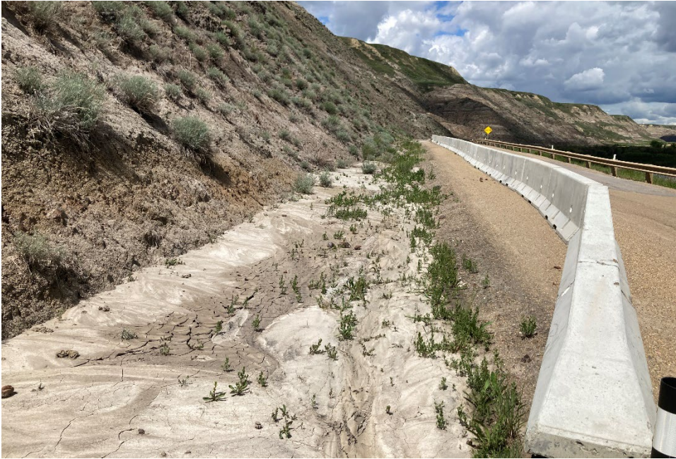
Photo 2 Failed material deposited into the west lane behind the jersey barriers, near the middle of the site, between the 2023 and 2024 inspections. Photo taken June 17, 2024, facing southeast.
