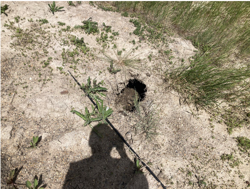
Photo 10 Sinkhole observed in the highway embankment slope downslope of C018-2. Photo taken June 18,2024, facing north.
