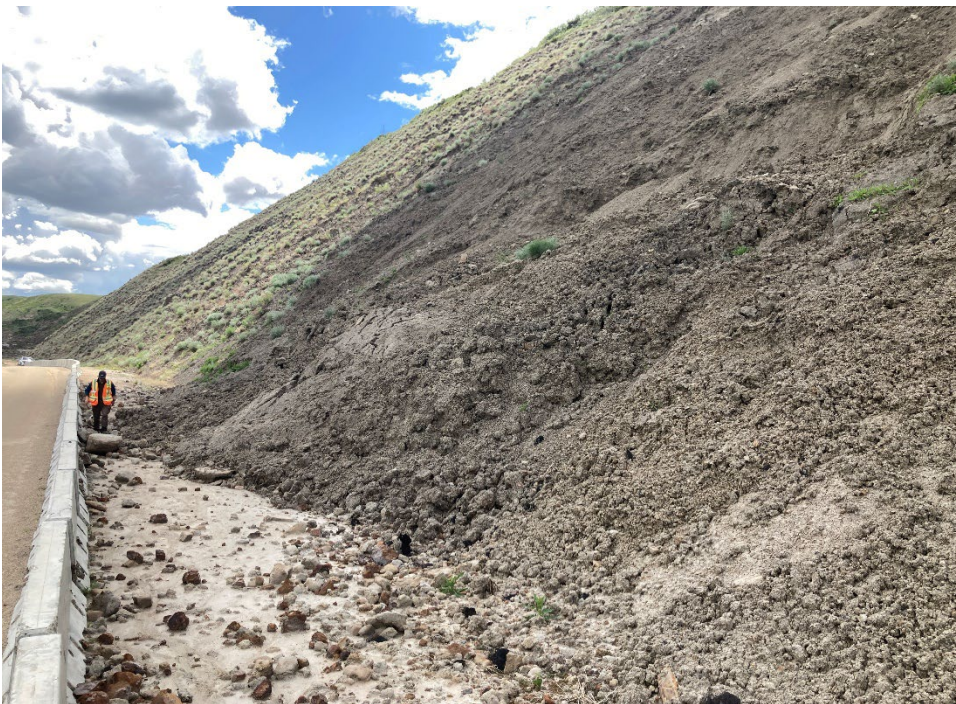
Photo 2 Failed material deposited into the west lane behind the jersey barriers, near the middle of the site, between the 2023 and 2024 inspections. Photo taken June 17, 2024, facing southeast.
