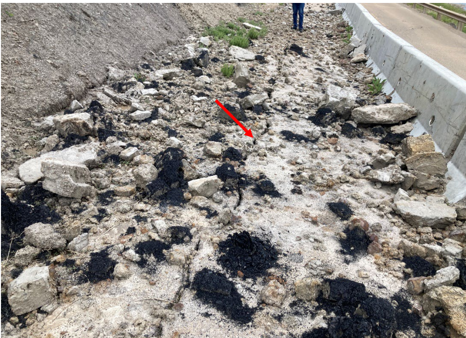
Photo 4 New pavement crack (approximately 25 mm wide and 20 m long, indicated by red arrow) that extends across both lanes near the northwest extent of the C018-2 site (northwest of the previous riverbank slide repair). Photo taken June 17, 2024, facing northwest.
