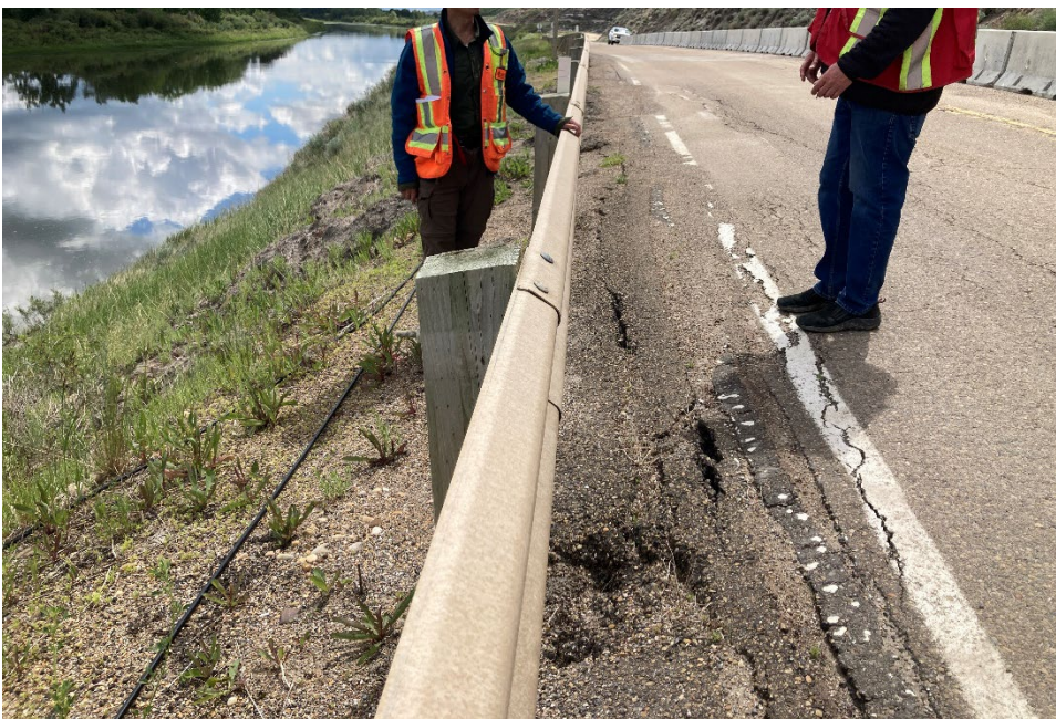
Photo 6 Pavement cracking at the edge of the east lane northwest of the C018-1 slide. Photo taken June 18, 2024 facing southeast.
