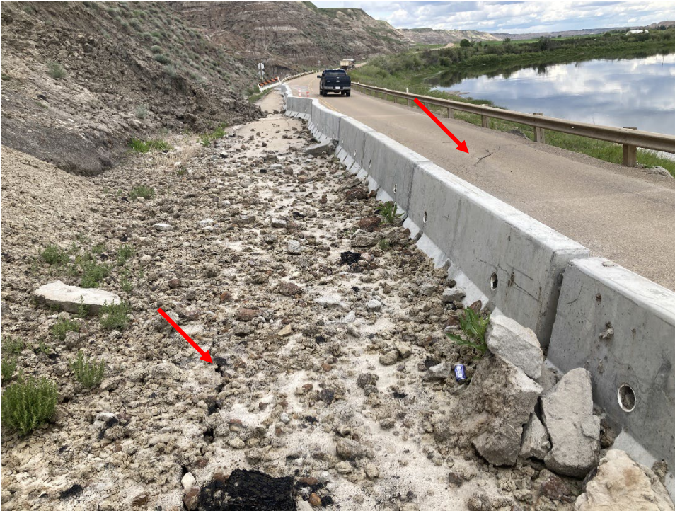
Photo 6 Pavement cracking at the edge of the east lane northwest of the C018-1 slide. Photo taken June 18, 2024 facing southeast.
