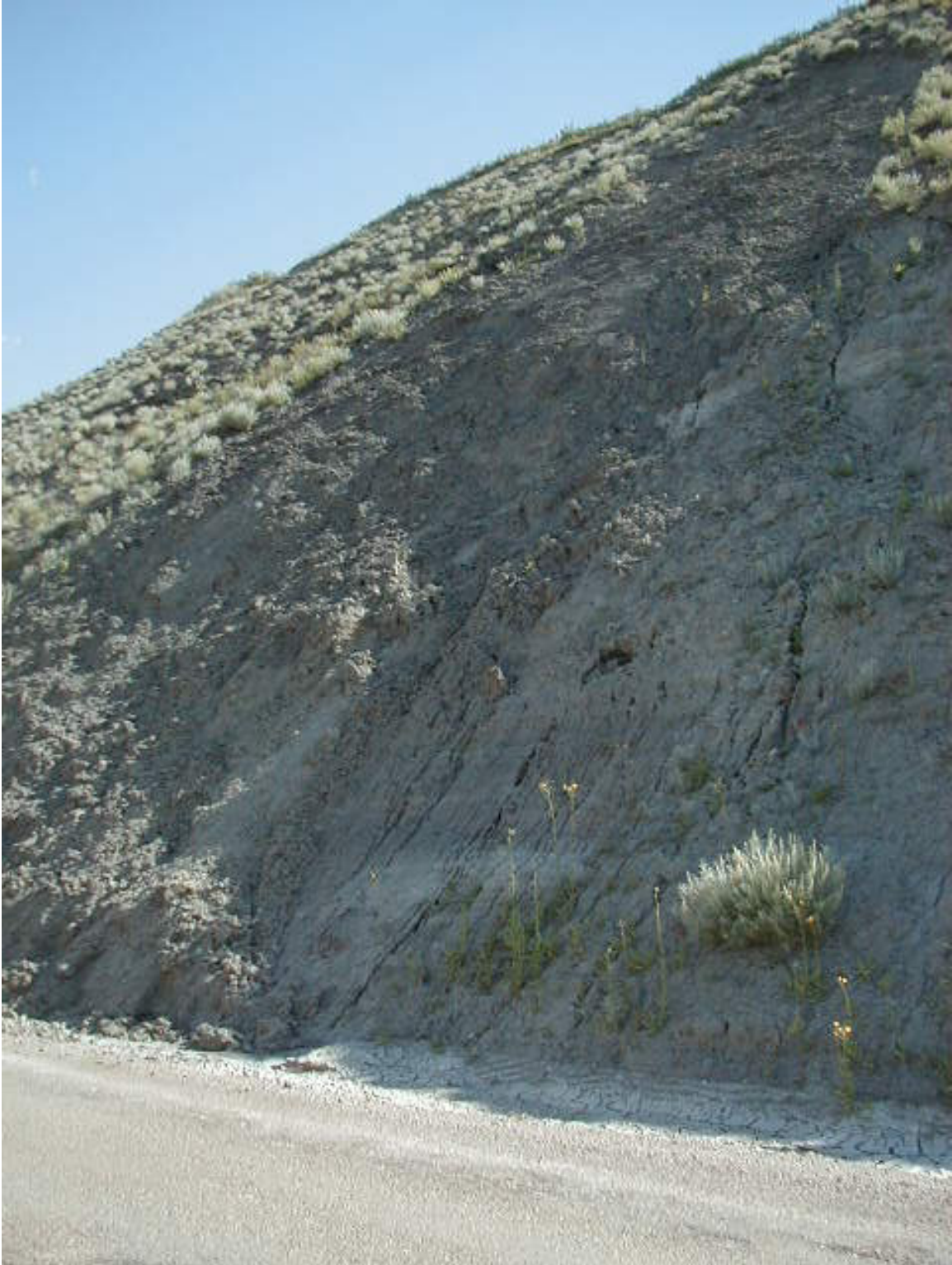
Backslope Erosion
