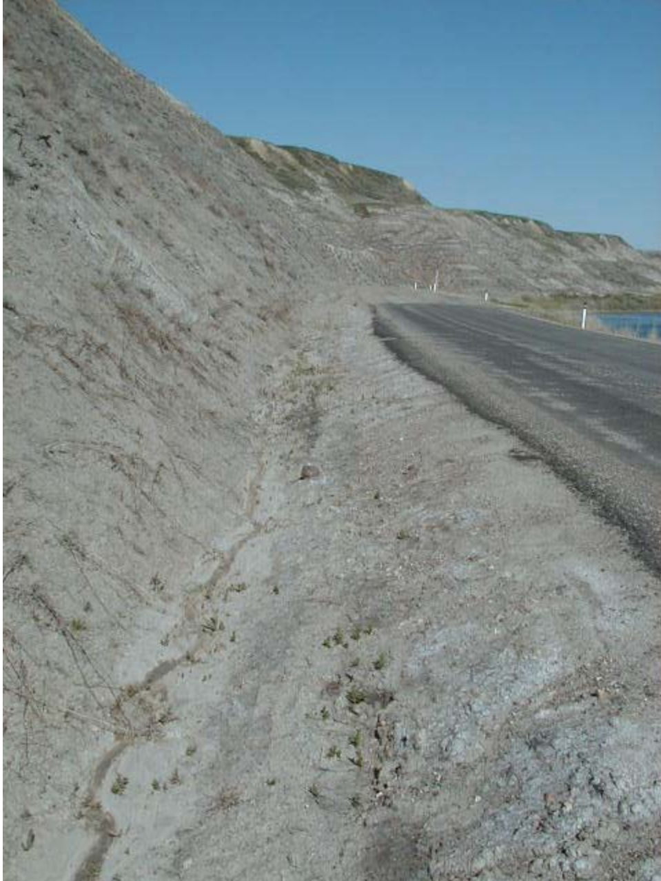
Well defined ditch on backslope side of highway
