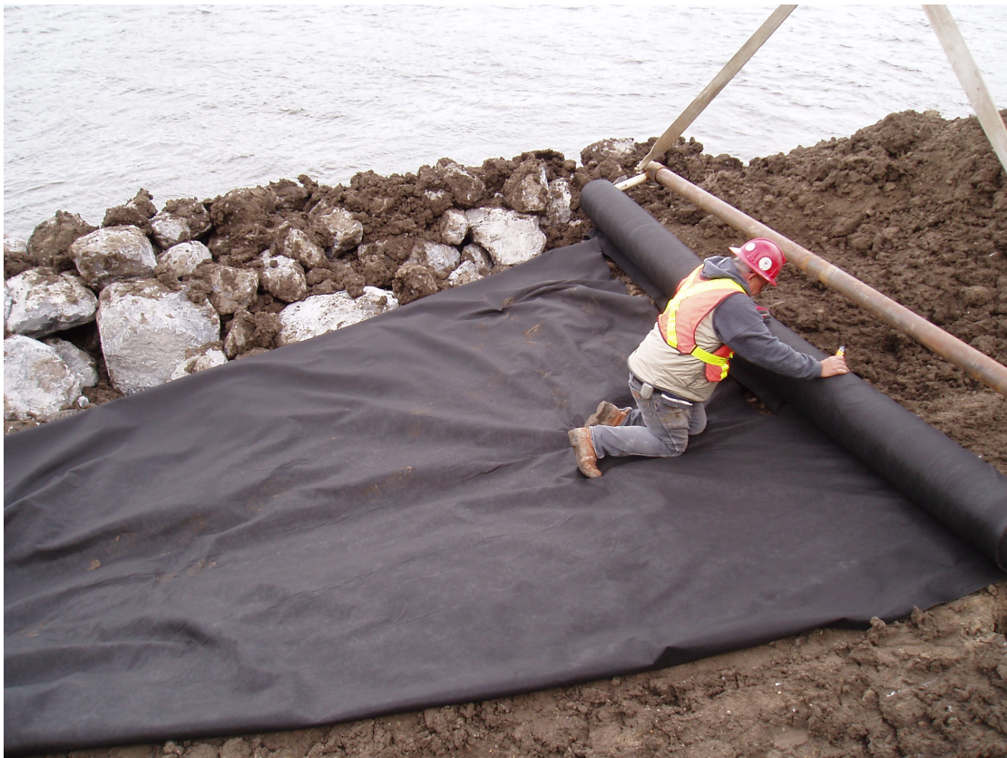
Placing rock riprap for berm.
