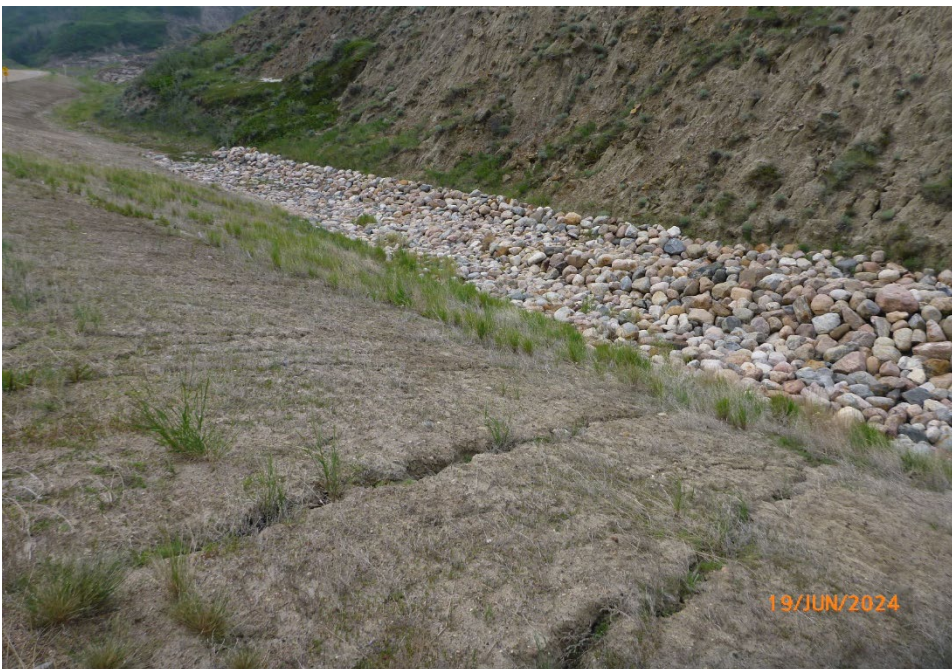
Photo 4 Riprap armouring downstream (south) of the gabion baskets. Photo taken June 19, 2024, facing south.
