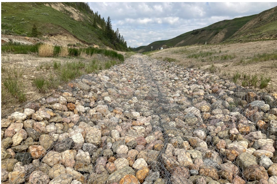
Photo 2 Gabion baskets were installed to achieve a channel shape and are performing well. Photo taken June 19, 2024, facing north.
