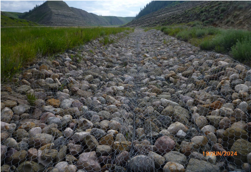
Photo 11 Gabions baskets installed in the south (eastbound) ditch east of the Morrin Bridge. Photo taken June 19, 2024, facing northwest.
