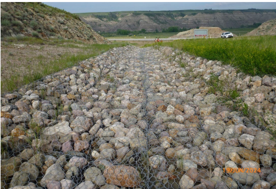
Photo 11 Gabions baskets installed in the south (eastbound) ditch east of the Morrin Bridge. Photo taken June 19, 2024, facing northwest.
