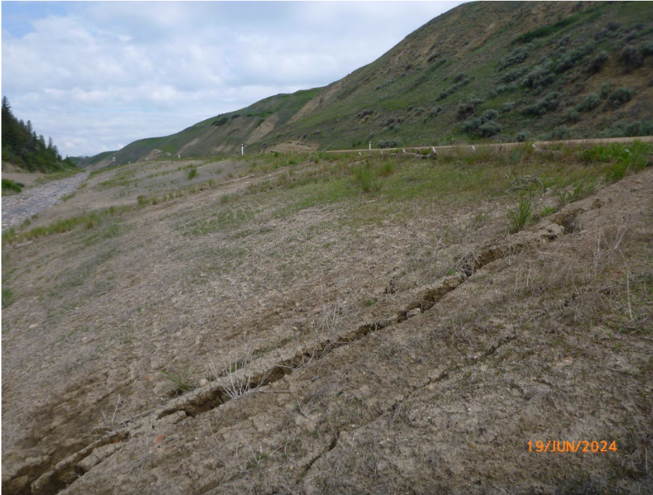
Photo 6 Minor erosion observed in the east (westbound) highway ditch. It appears as though the ditch was previously repaired with a rolled erosion control product. Photo taken June 19, 2024, facing north.
