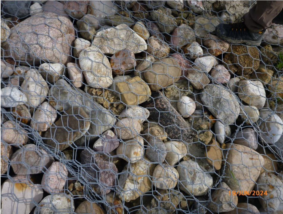
Photo 4 Riprap armouring downstream (south) of the gabion baskets. Photo taken June 19, 2024, facing south.
