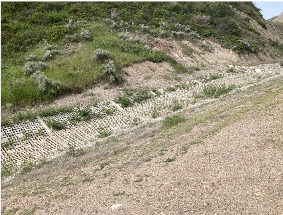
Photo 8 Length of ditch repaired using articulated concrete blocks. Photo taken June 19, 2024, facing southwest.
