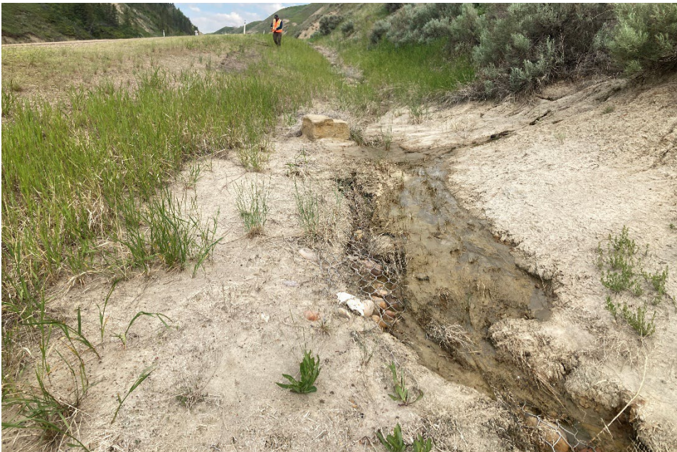
Photo 6 Minor erosion observed in the east (westbound) highway ditch. It appears as though the ditch was previously repaired with a rolled erosion control product. Photo taken June 19, 2024, facing north.
