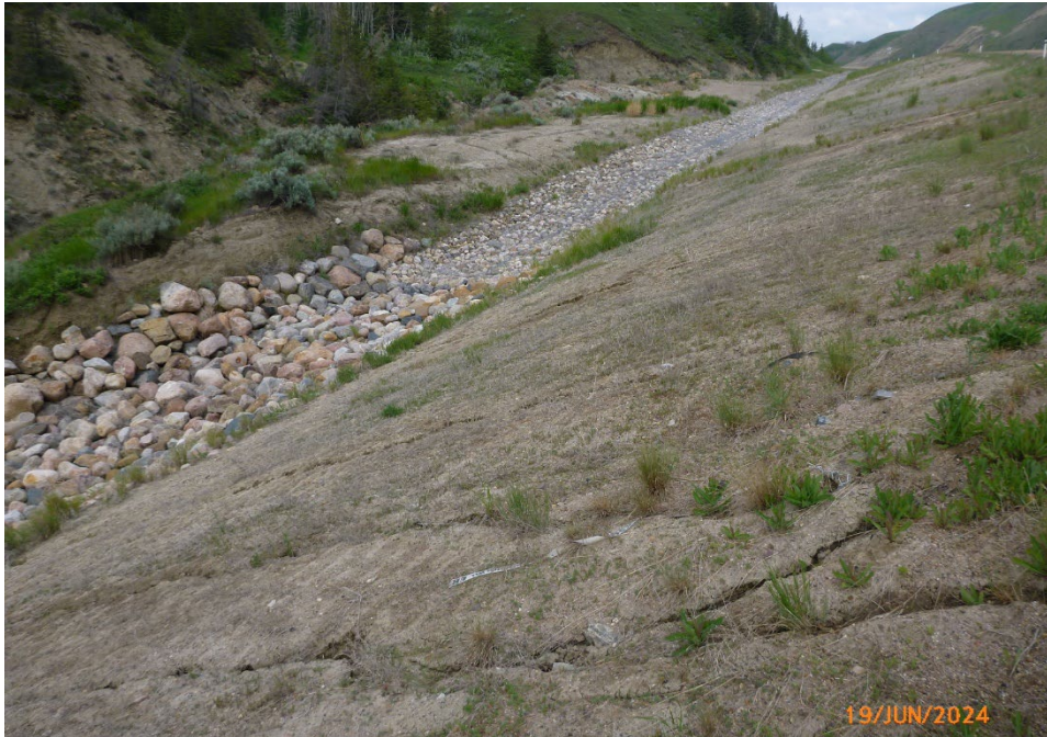
Photo 2 Gabion baskets were installed to achieve a channel shape and are performing well. Photo taken June 19, 2024, facing north.
