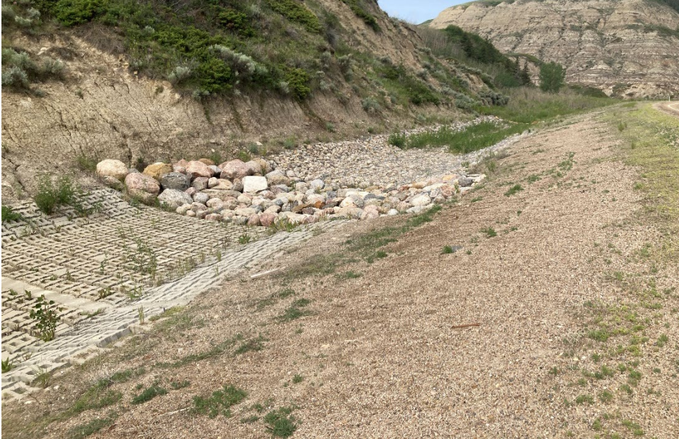
Photo 8 Length of ditch repaired using articulated concrete blocks. Photo taken June 19, 2024, facing southwest.
