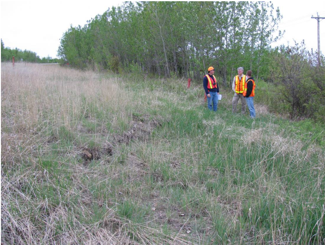
Photo #7 Active scarp crack downslope of the wall, looking west
