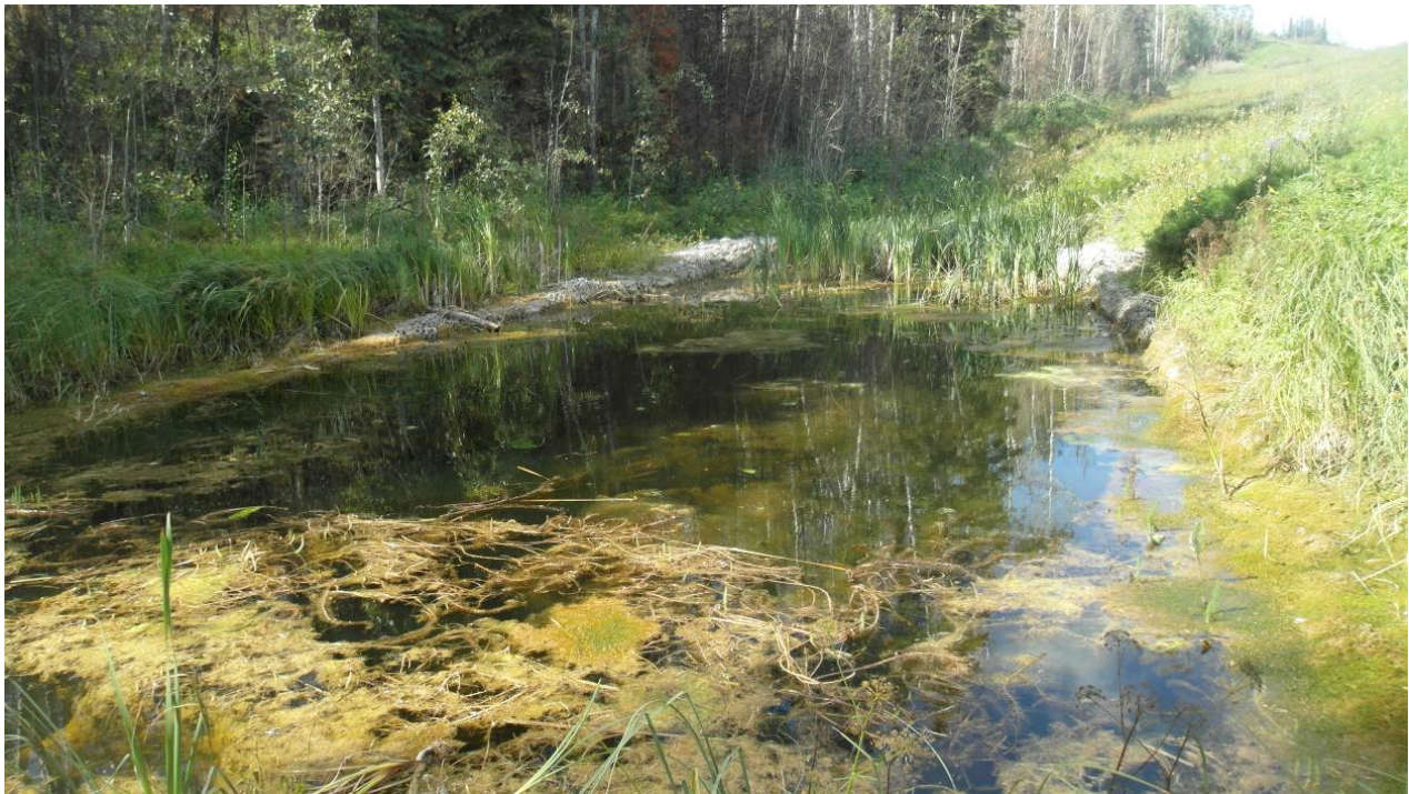
Photo #8 - Looking north at the stilling pond
