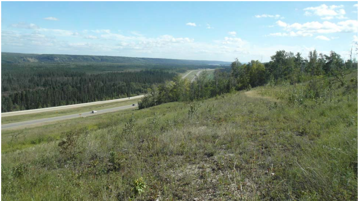
Photo #13A - Looking north at the third bench of the west back slope; seepage was noted within the northern limit of the bench.
