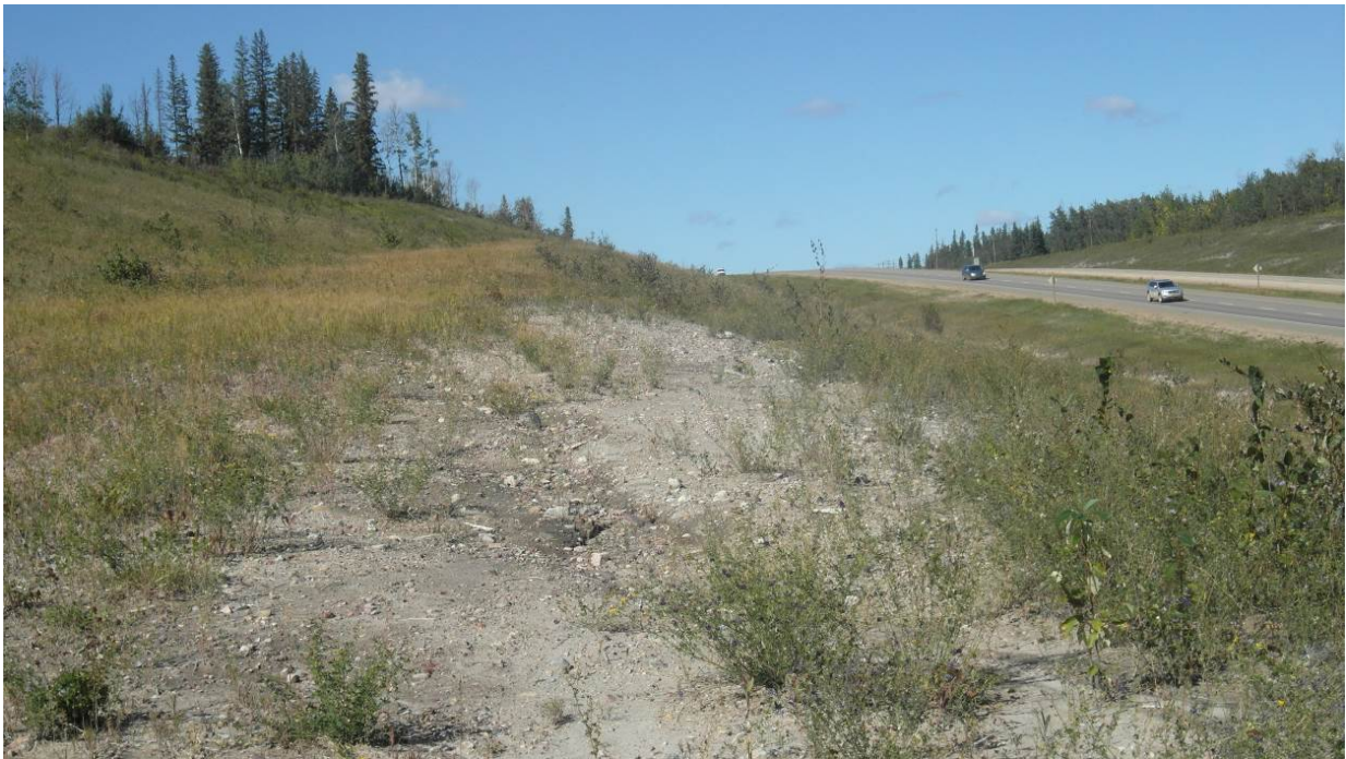
Photo #12 - Looking north at the first bench of the west back slope; dry bench with spots bare of vegetation.
