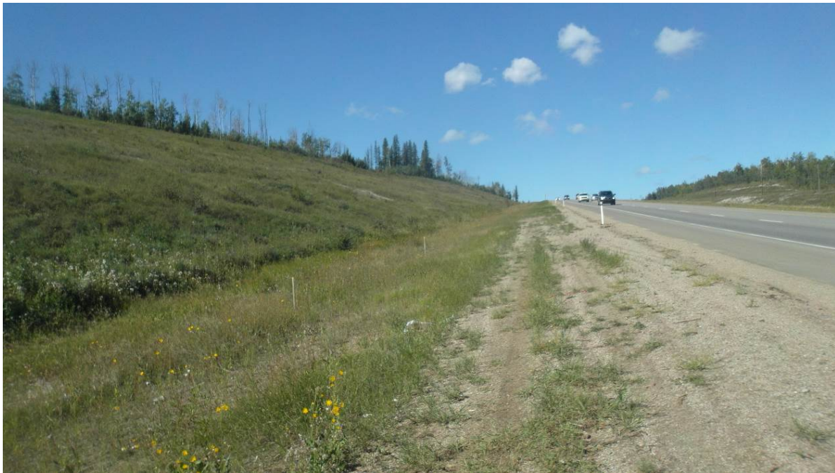
Photo #10 - Looking north along the toe of the highway west back slope; note the absence of vegetation within a strip of the highway side slope.
