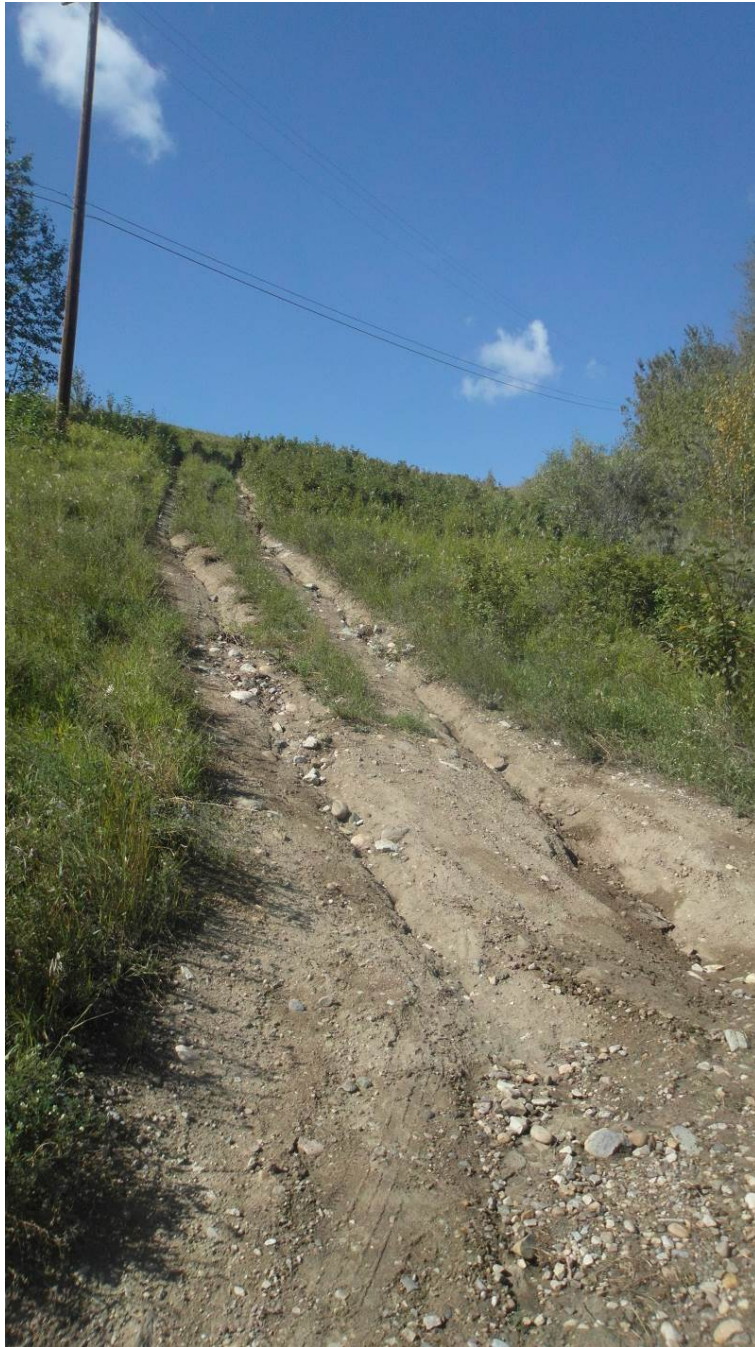
Photo #1A - Looking northwest at a strip bare of vegetation within the east side slope; note the presence of erosion rills on the exposed slope surface.
