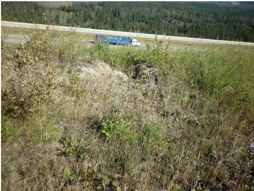
Photo #19 - Looking east at old erosion rill covered with grass vegetation.
