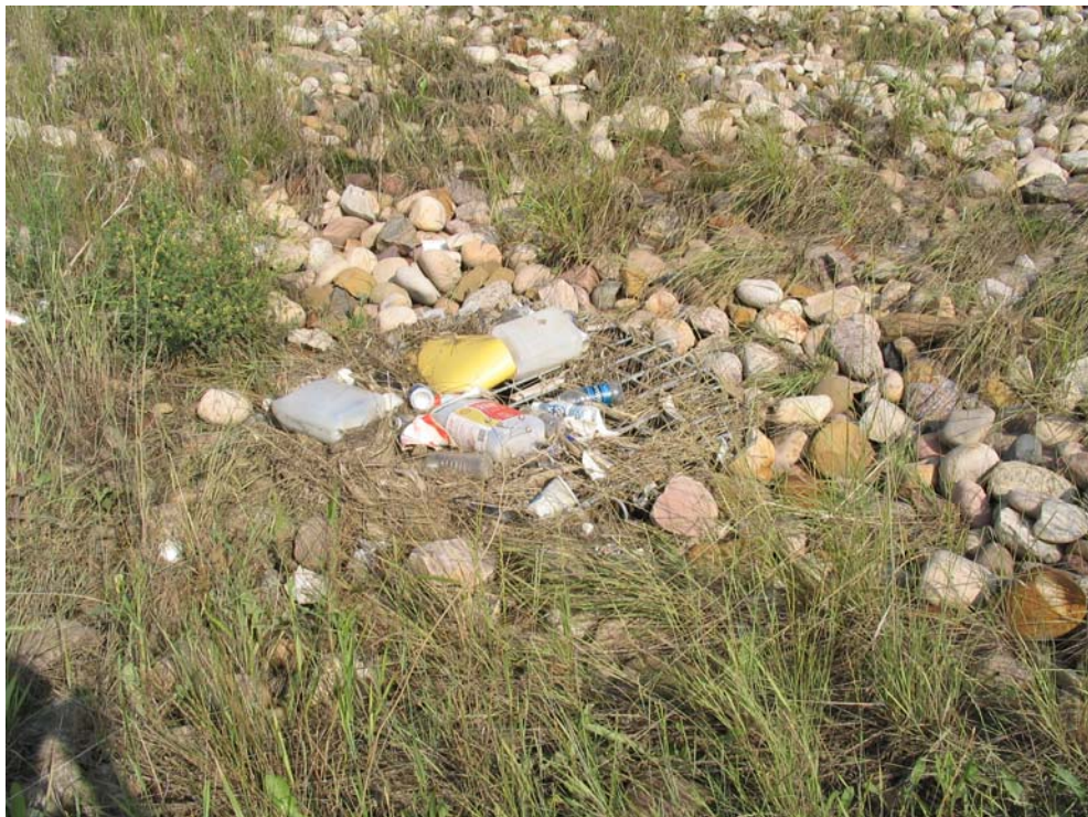
Photo 6 Drop Pipe Grate Needs to be Cleaned.
