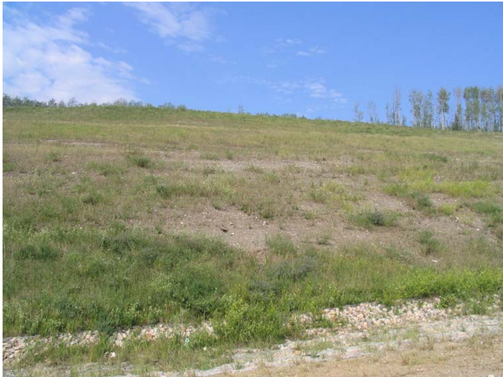
Photo 12 - Bare Area on Lower Part of Backslope.
