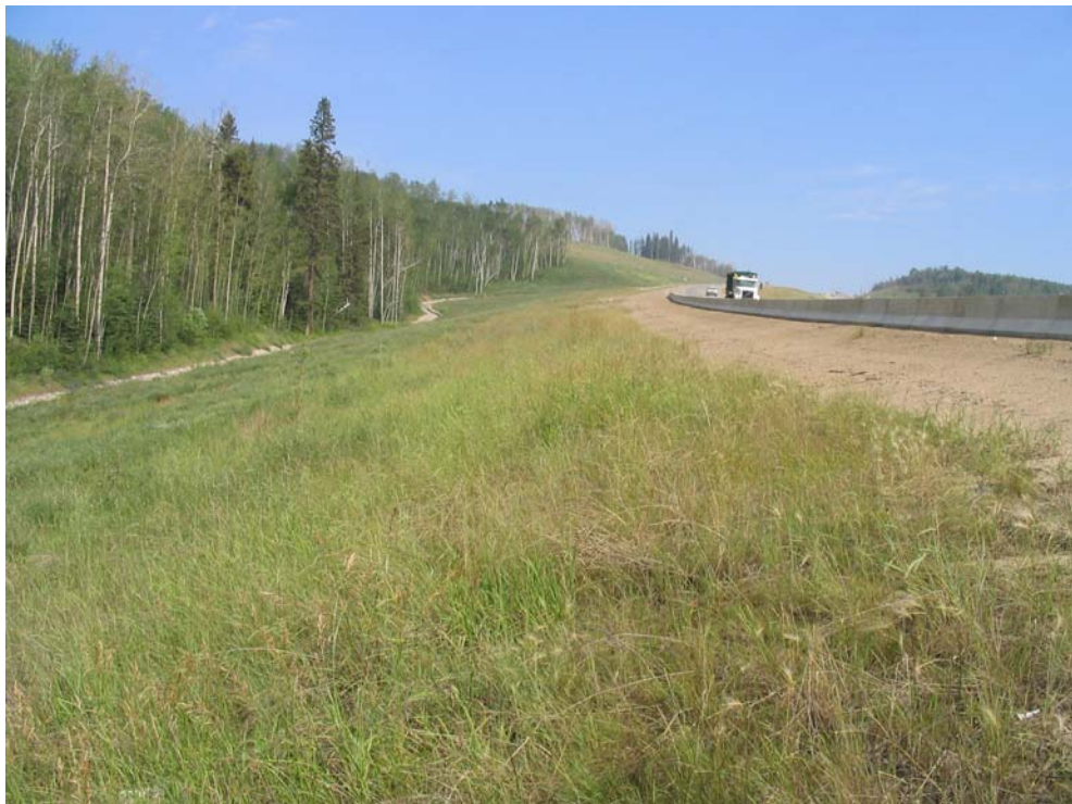
Photo 8 - Looking North along West Sideslope from South End.
