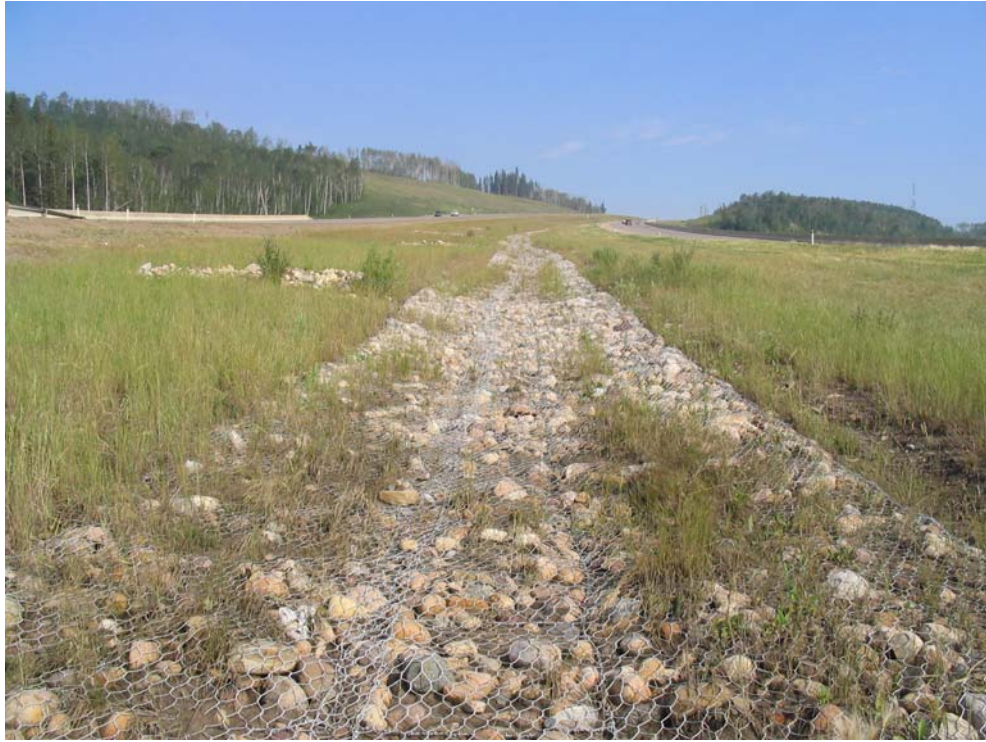
Photo 7 - Gabions in Median Ditch.
