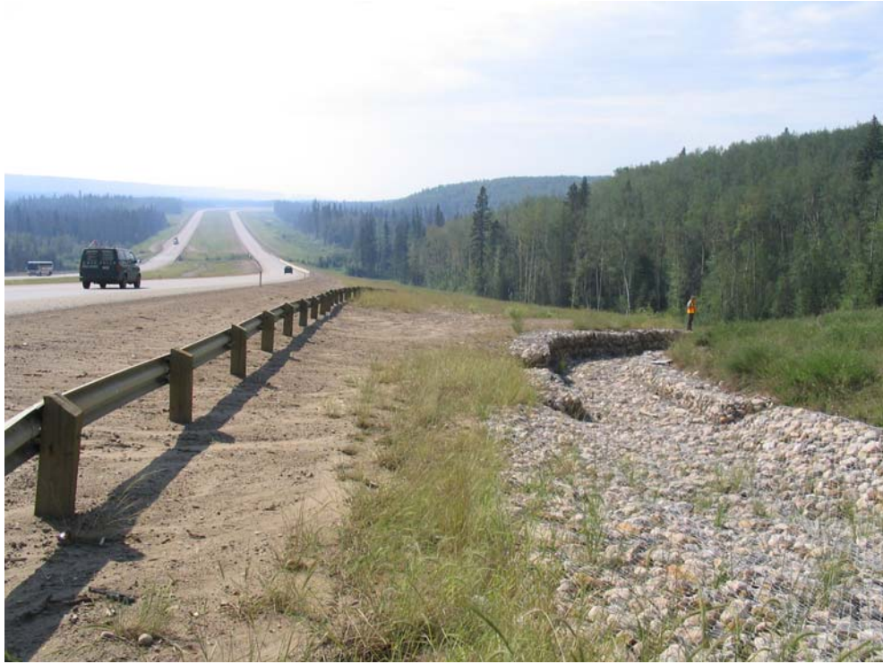
Photo 9 - Looking South along West Sideslope from North End.
