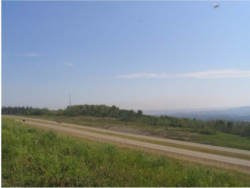
Photo 13 - Bare Backslope on East Side of Highway at North End of Site.
