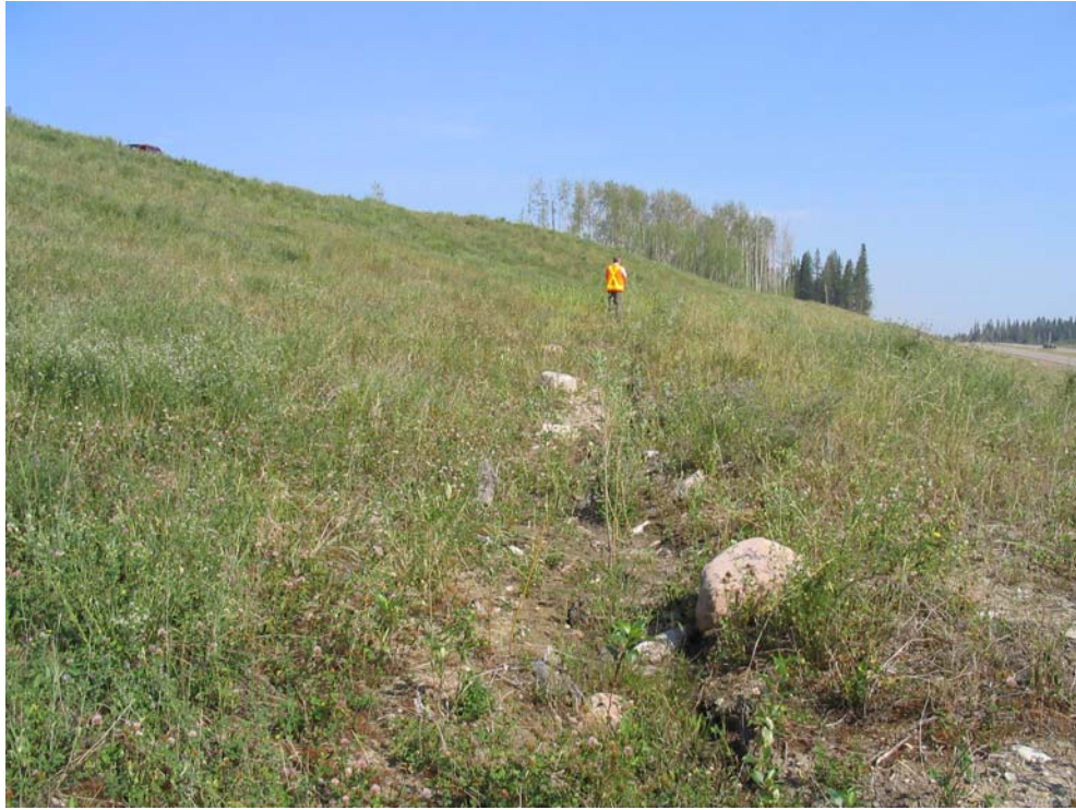
Photo 11 -Third Bench of High Backslope.
