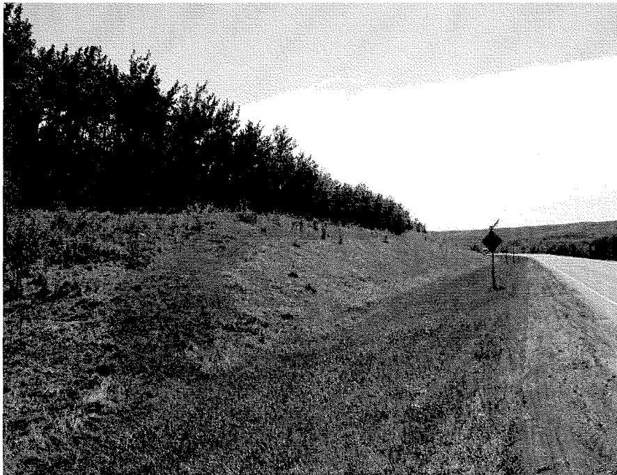
Photo 4 - Looking south at the highway backslope and east side slope
