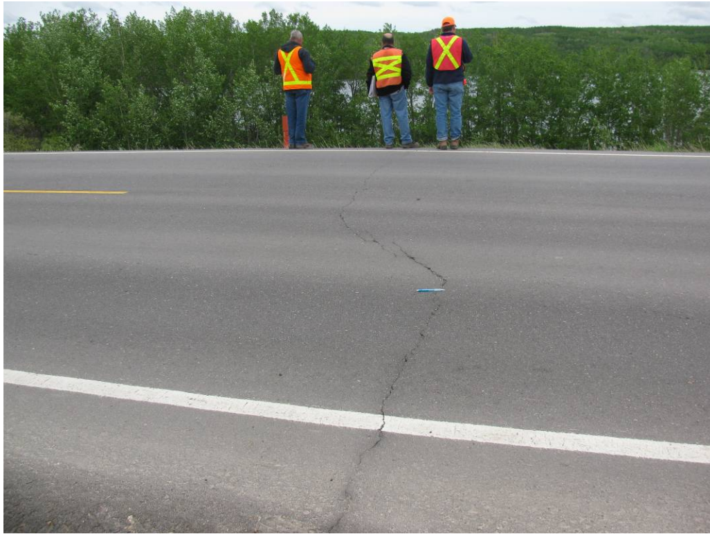
Photo #5 Transverse reflective crack at the southern limit of the slide area (looking west)
