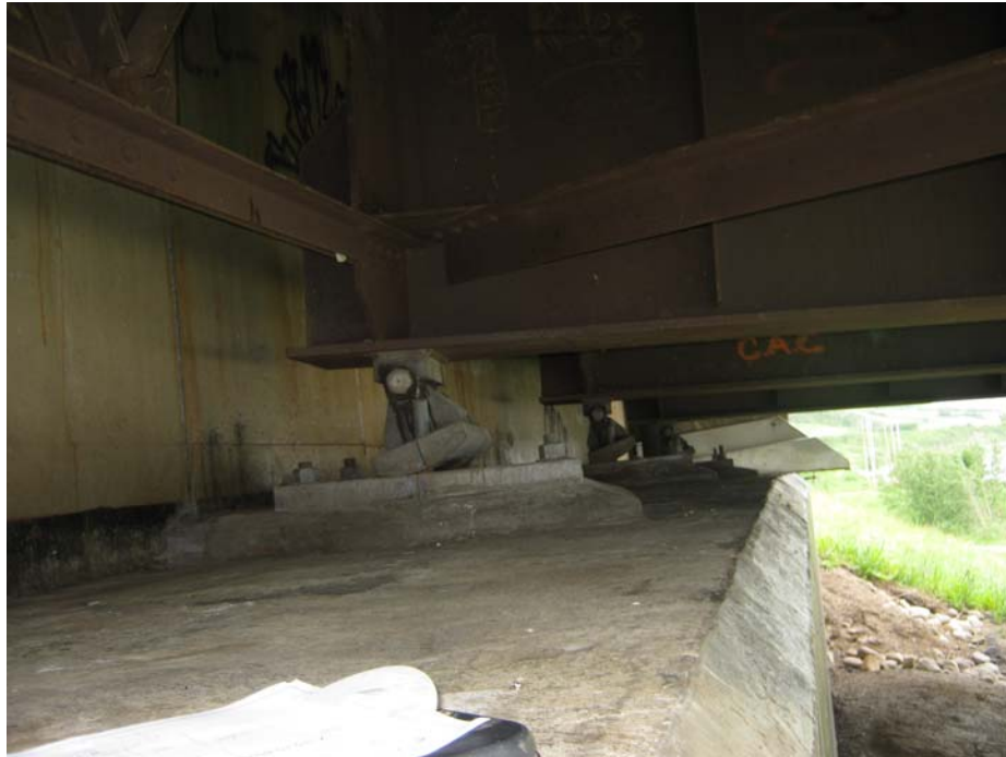
Photo#5 Looking east at the steel girder rocker bearings
