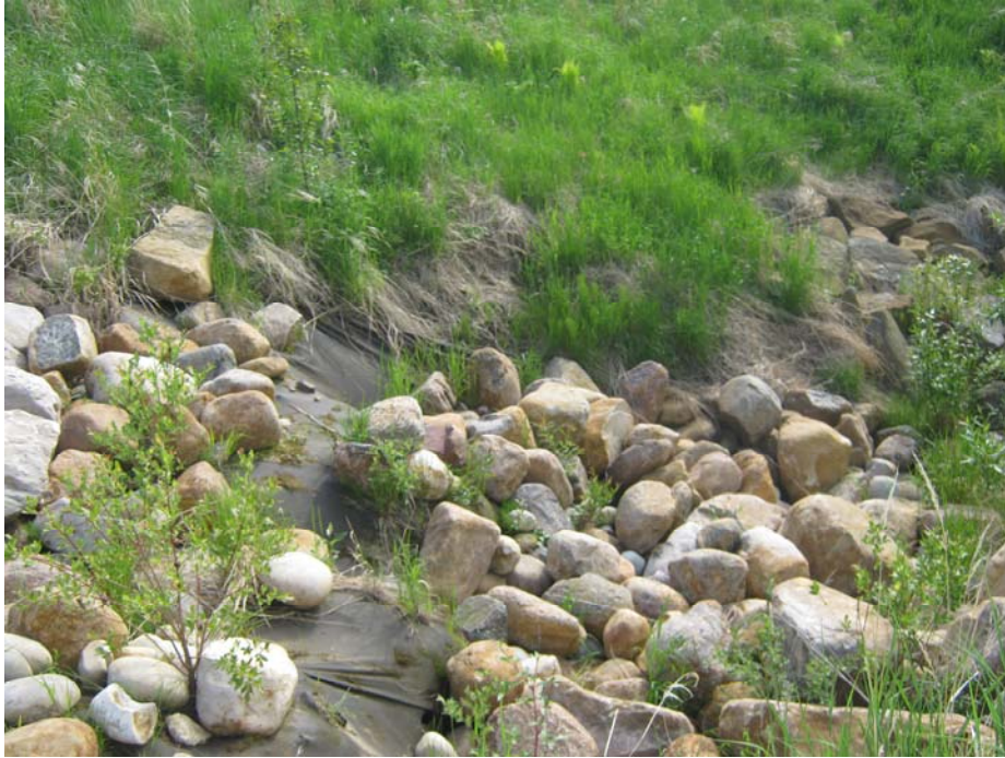
Photo#5 Exposed non-woven geotextile fabric below heavy rock riprap (looking south)
