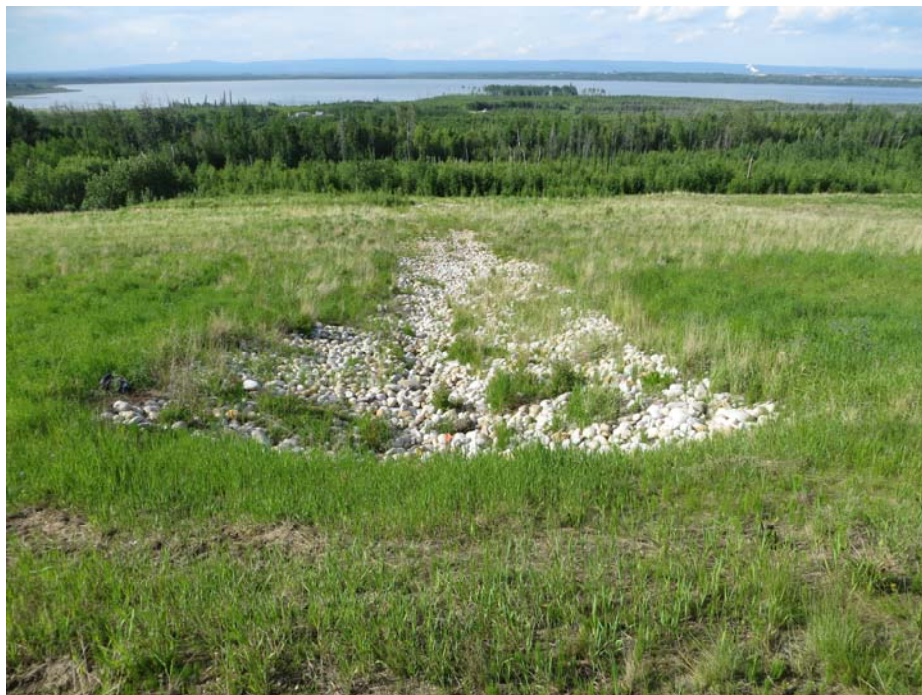
Photo#4 Looking towards the riprap-lined swale from the crest of the slope (looking west)
