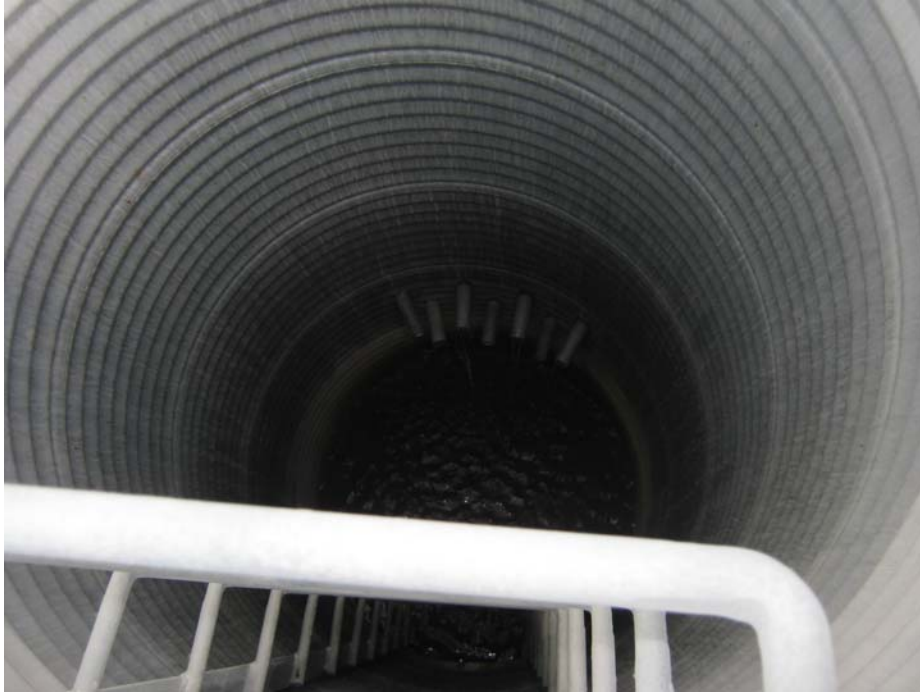
Photo#7 Looking inside the drainage collection manhole
