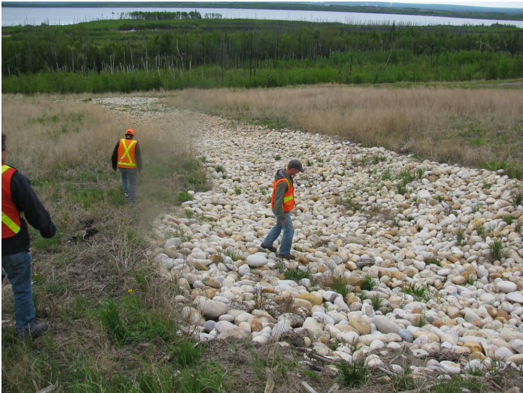
Photo#3 Looking towards the riprap-lined swale from the crest of the slope (looking west)
