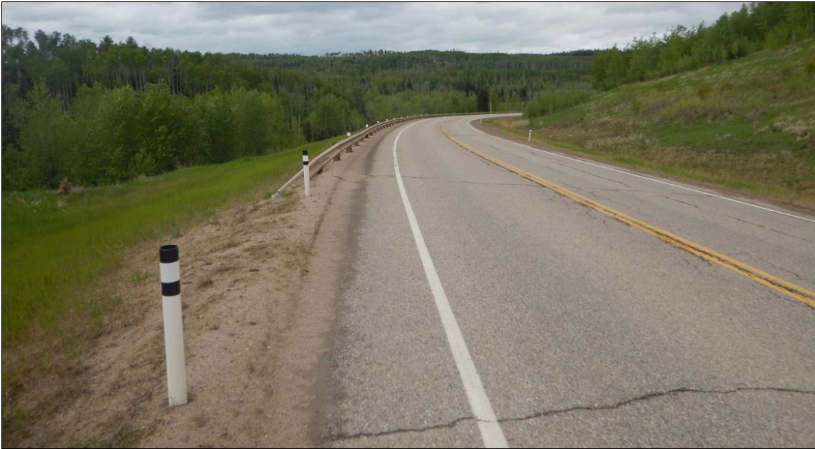
Photo No.1 - Looking north from the southern limit of the site at transverse and longitudinal cracks on the highway
