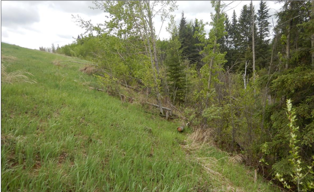
Photo No.11 – Tilting trees and deadfall downslope of the most distressed area on the highway surface (i.e. location of old slump above creek channel).
