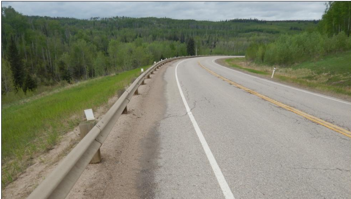
Photo No.2 - Looking north from the southern limit of the site at diagonal Crack A
