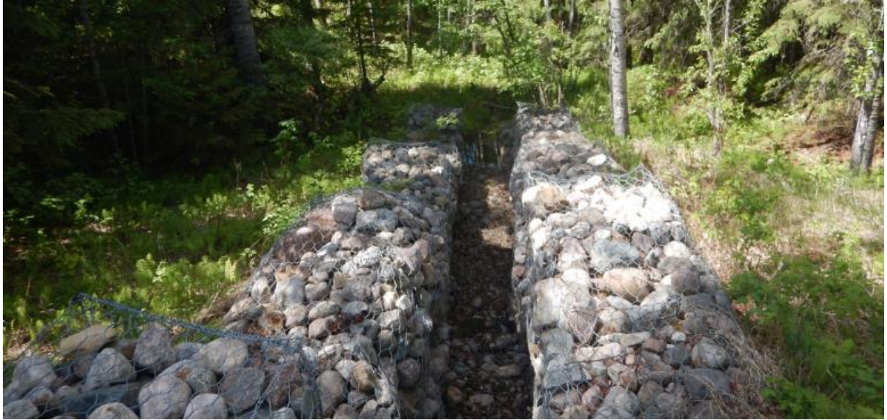
Photo No.9 - Looking west at the gabion basket channel
