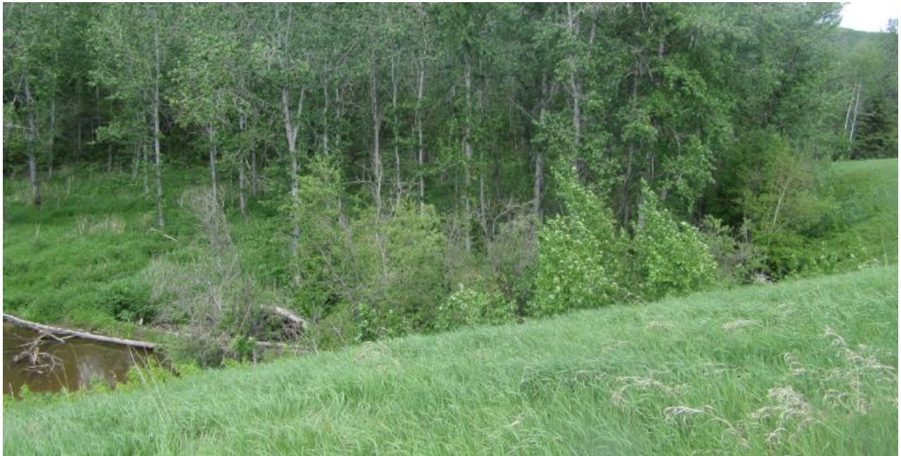
Photo No.10 – Looking west at an old slump above Beaver Dam 2
