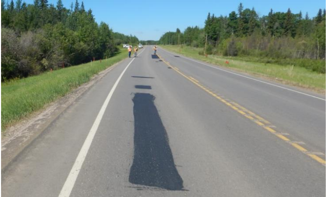
Photo No.3 - Looking west from the eastern flank of the EBL landslide (NC58) at the 2019 crack seals
