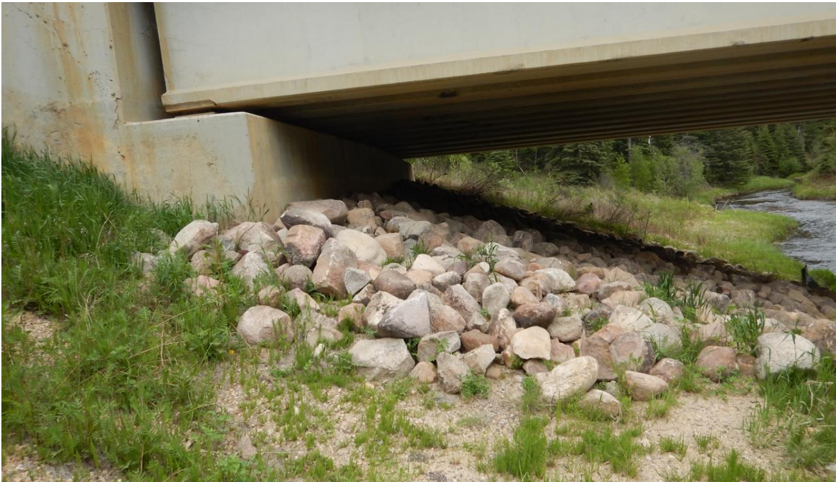
Photo No. 2 – North Abutment (Looking East) showing riprap placed by AT in 2021
