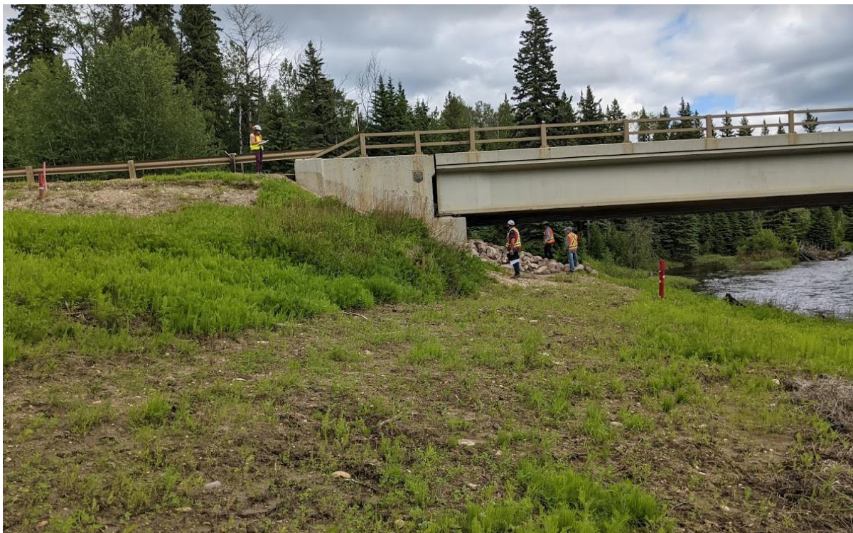
Photon No. 6 –Looking east at the NW approach fill headslope
