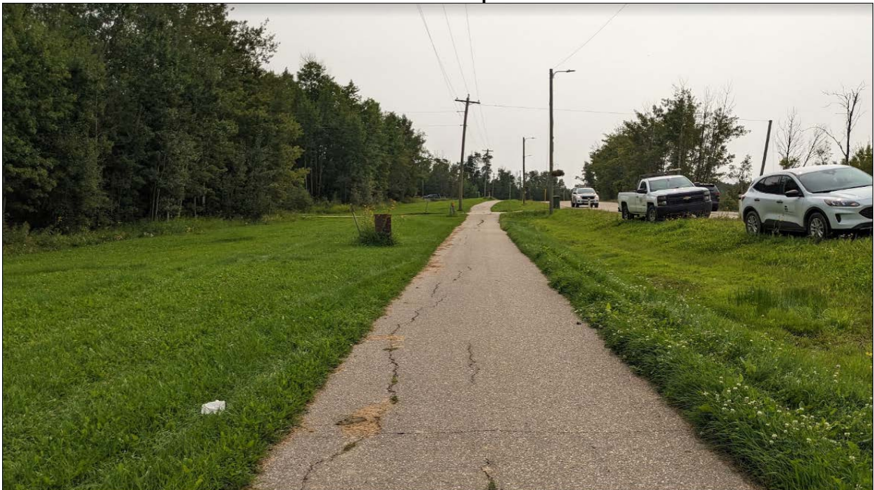
Photo 6. Pedway on the east side of the highway. Note Power Pole No. 2 and Anchor Pole No. 3 tilting due to the landslide movement.
