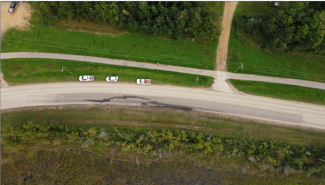
Aerial Photo 8. Landslide impacting approximately 80 m of highway surface extending from the recent ACP patch placed on the northern flank of the slide to south of Power Pole No. 2 as shown within the black arrows. Note ponding water west of the treed area (bottom part of the photo).
