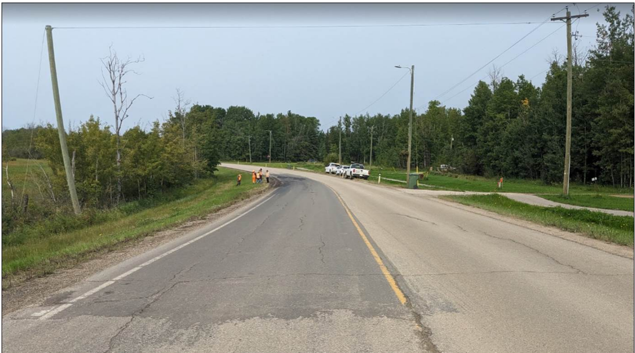
Photo 2. Looking north at the landslide area. Anchor Power Pole No. 3 on the LHS and the Power Pole No. 2 on the RHS of the photo are bent due to the high tension in the overhead cable.
