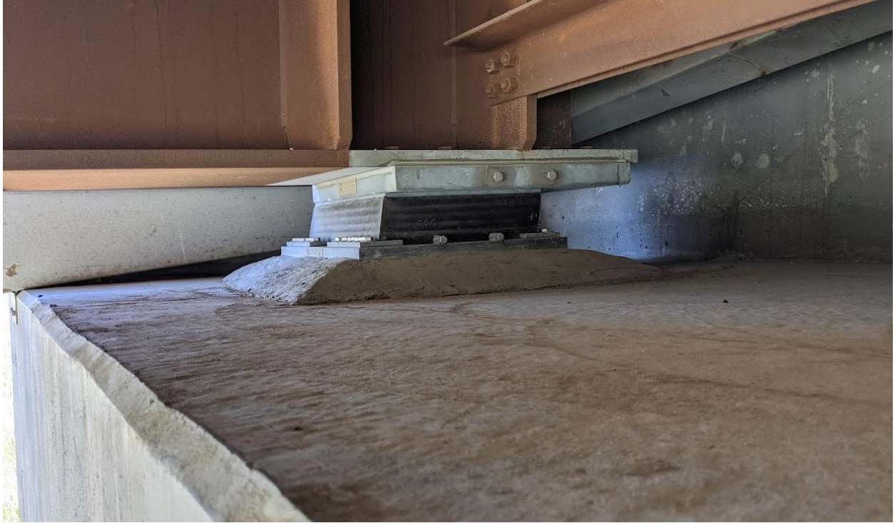
Photo 6 – Bridge bearing position appears be in conformance with design drawings
