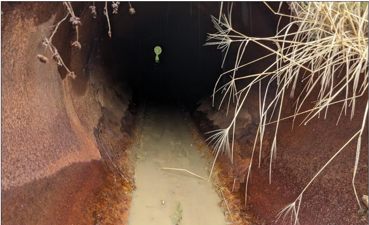
Photo 10. Looking inside culvert C3 outlet.
