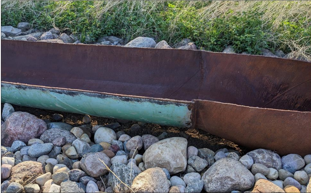
Photo 11. Outlet of culvert C3, installed in 2021. There is a void below the half pipe extension piece.
