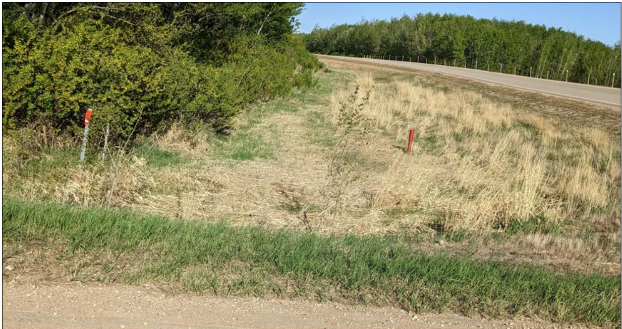
Photo 2. Highway's north ditch to the east of the approach.
