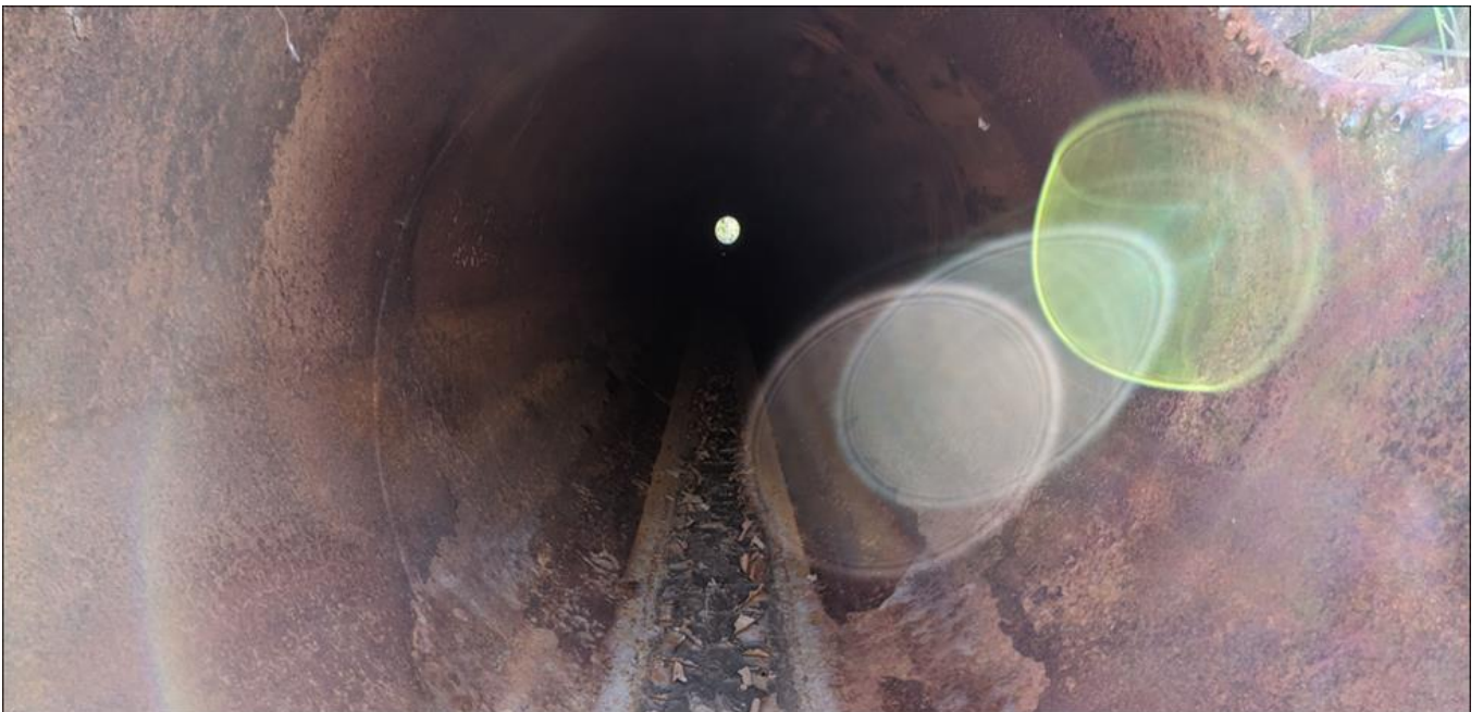
Photo 10. Looking inside culvert C3 outlet.
