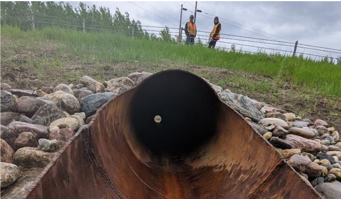
Photo No.8 – Looking inside new culvert C3 outlet.
