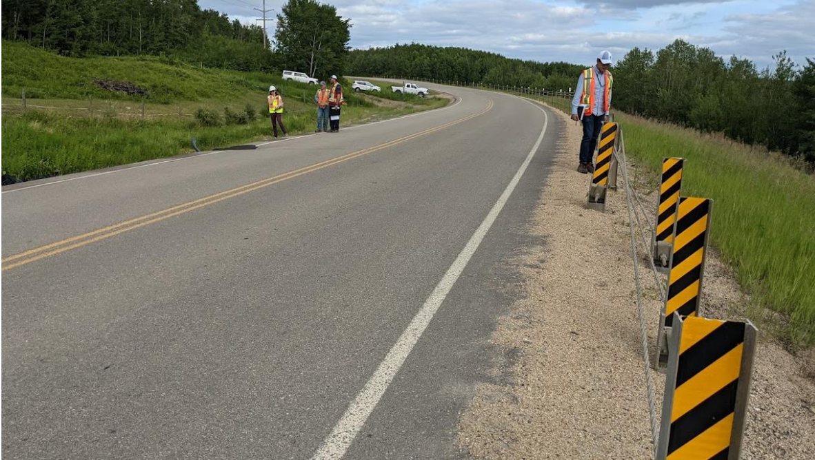
Photo No. 1 – Looking at the highway surface from the western limit of the site
