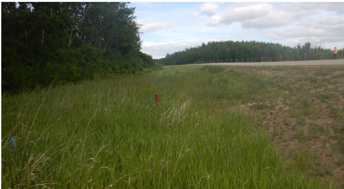
Photo No. 2 – Looking east at highway north ditch to the east of the approach; scarce vegetation on the highway side slope
