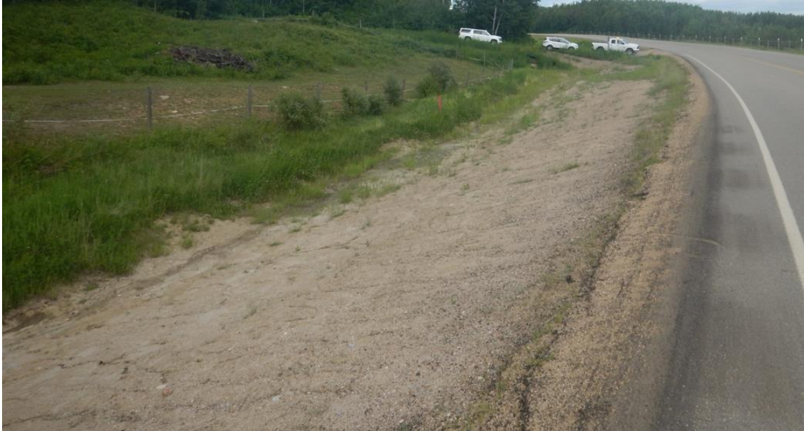
Photo No. 5 – Looking east at ditch regraded in 2019 by WSP; the north ditch has been regraded from culvert C1 outlet to culvert C3 inlet; culvert C2 appears to have been abandoned; side slopes and sections of the ditch are bare of vegetation
