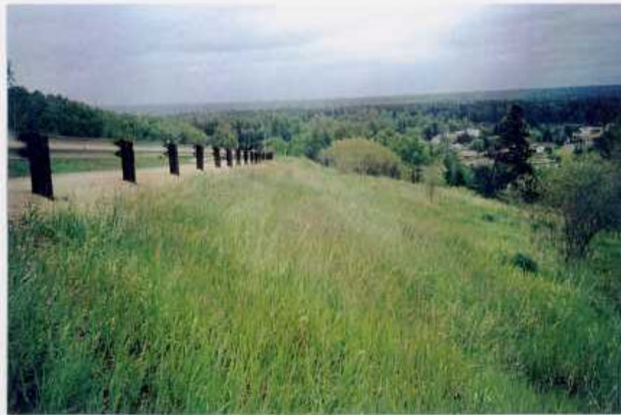
PHOTO NC14-4 LOOKING SOUTHEAST AT POSSIBLE GRABEN AREA IN UPPER SLOPE.
