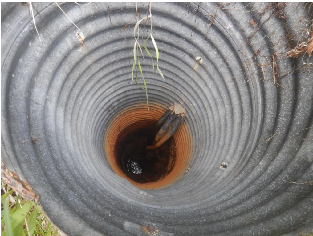
Photo No. 10 – Looking inside MH2
