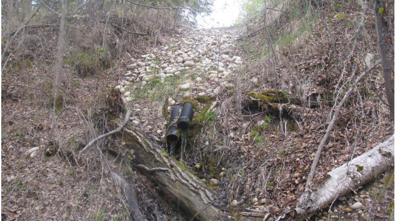
Photo #12 Subdrain Outlets. Note heavy flow from the HDPE pipes
