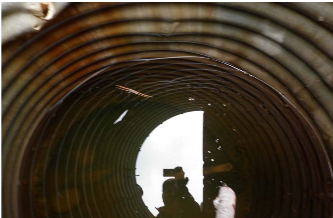
Photo #2 Standing clear water inside MH#1
