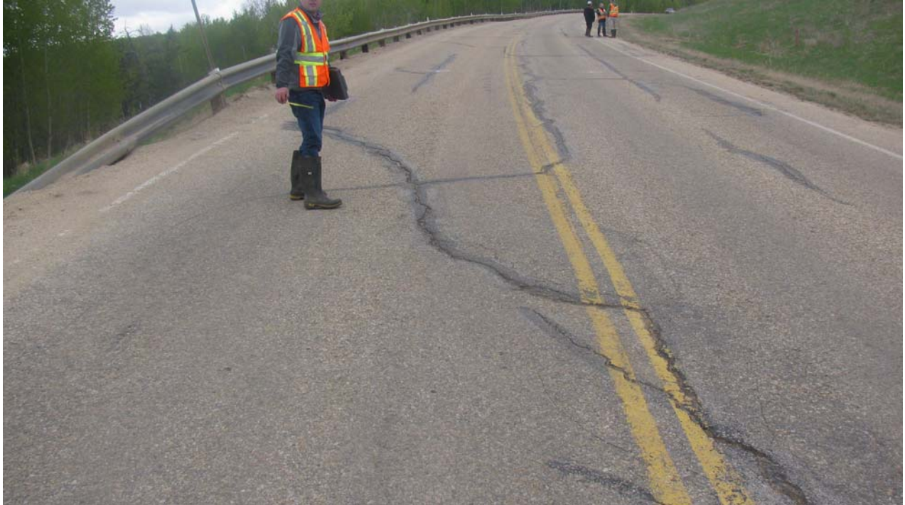
Photo #7 Open arc-shaped crack at the northern limit of Mid-Hill slope section (Looking northwest)
