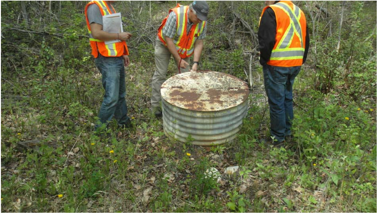
Photo #1 Looking at the area located upslope of drainage collection manhole #1
