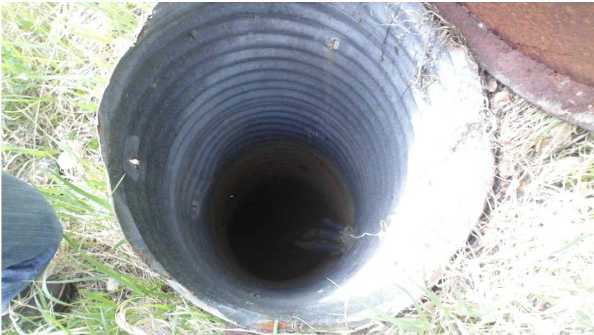
Photo #12 Looking inside MH#2
