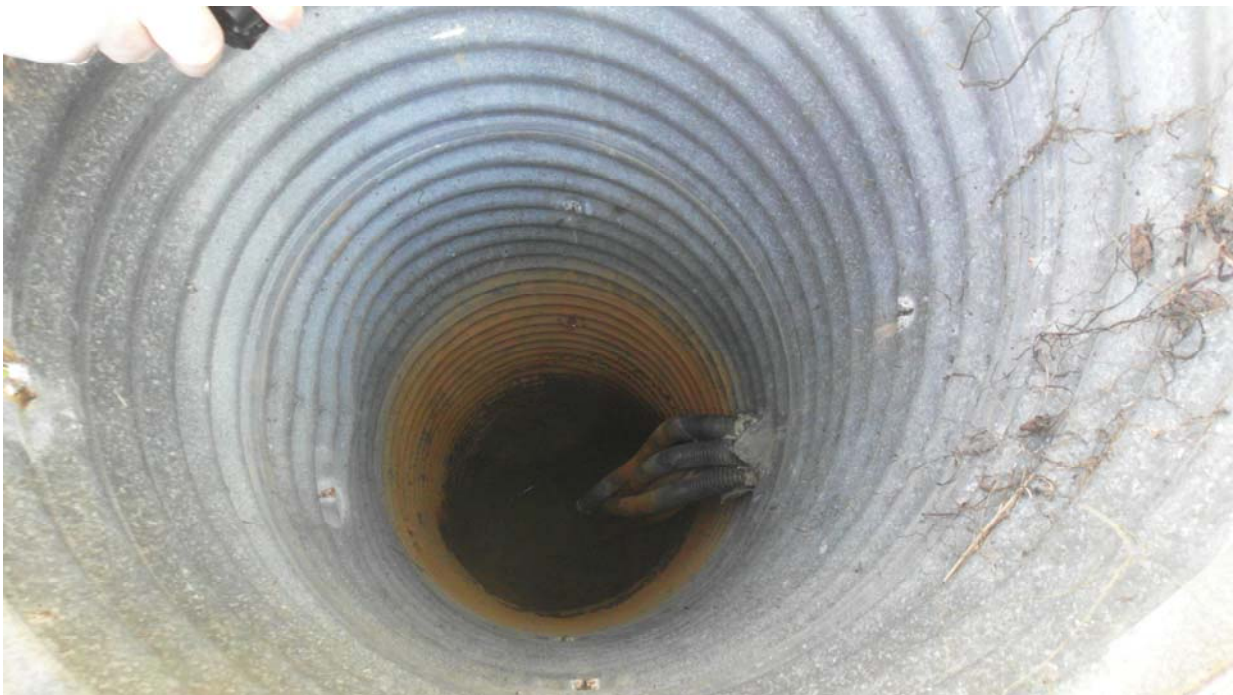
Photo #10 Looking inside MH#2
