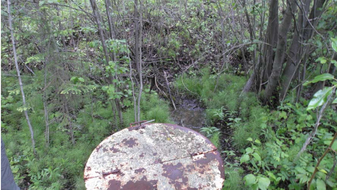
Photo #1 Looking at natural gully located upslope of drainage collection manhole #1
