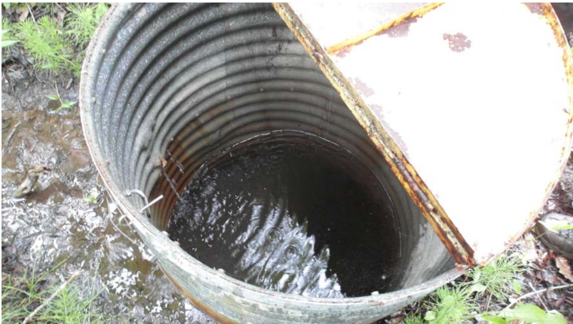
Photo #2 Standing water inside MH#1; note that the drain outlets are completely submerged under water
