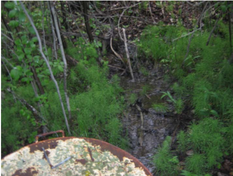
Photo #1 Some water around the Uphill CSP drainage collection manhole (MH#1)
