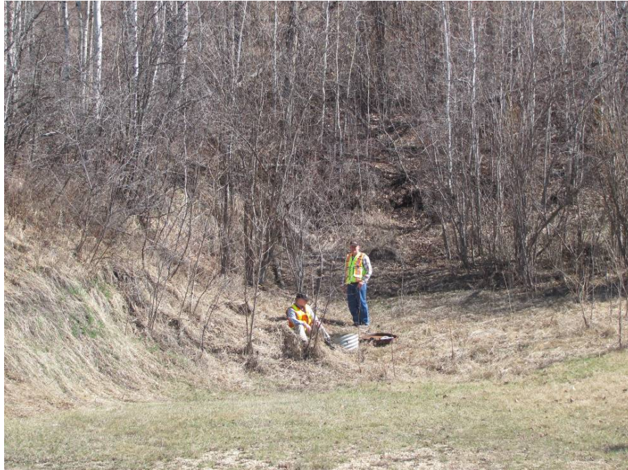
Photo #5 Looking east at MH#2 from the bottom of the slope; note the presence of a local old slump above the manhole location
