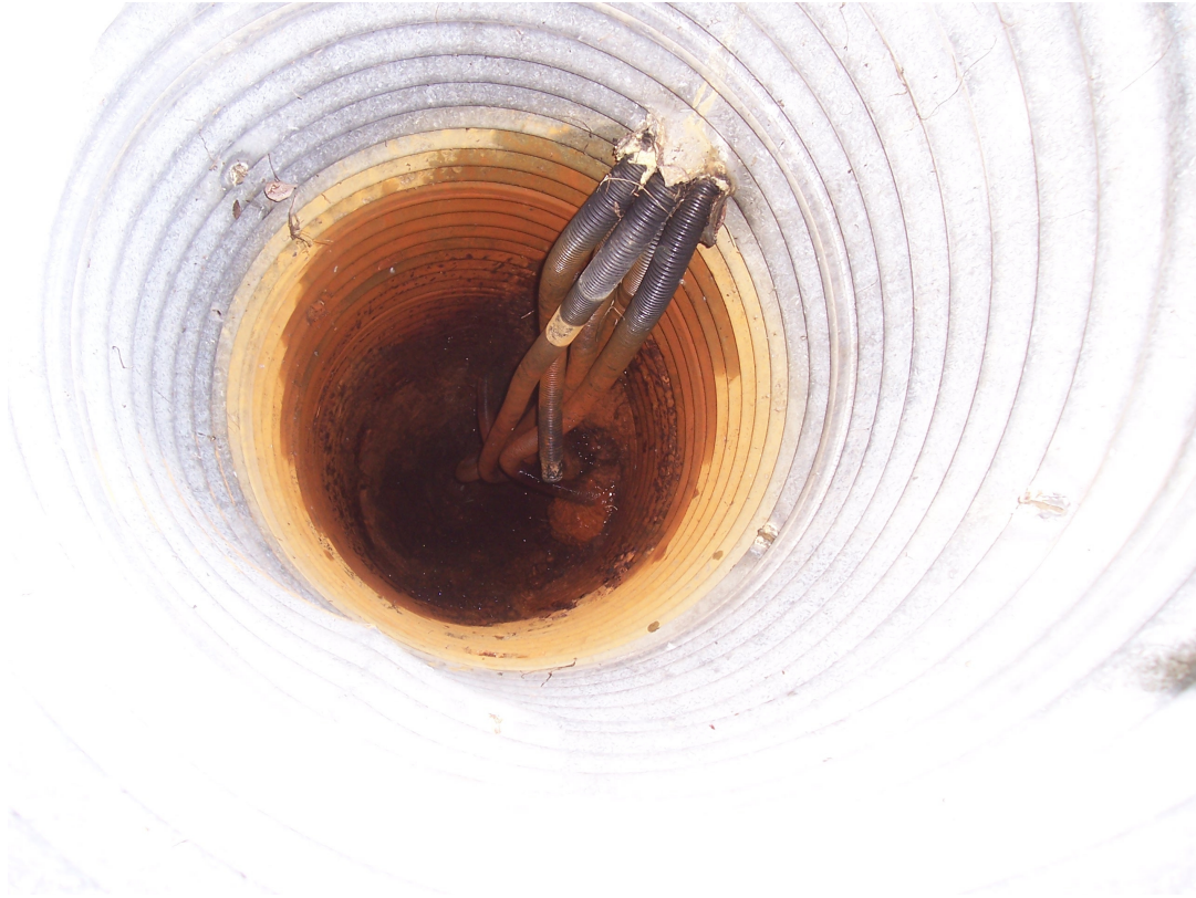
Photo #7 Looking inside the downhill drainage collection manhole (MH#2)
