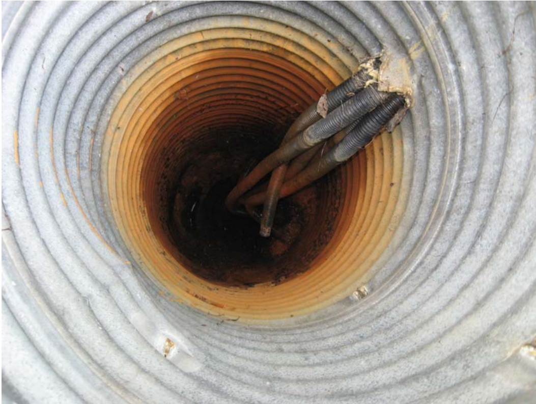
Photo 3 Collection point at the toe of the slope.
