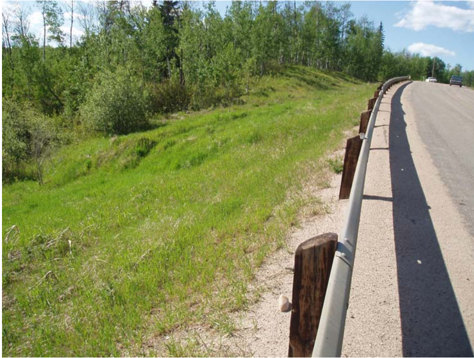
Photo 3 Scarp and graben feature on the sideslope unchanged.
