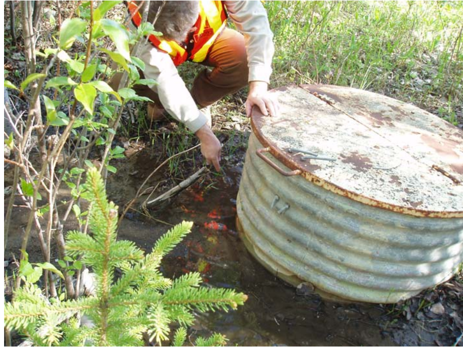
Photo 5 Backslope collection point, Cleaning the surface drainage holes
